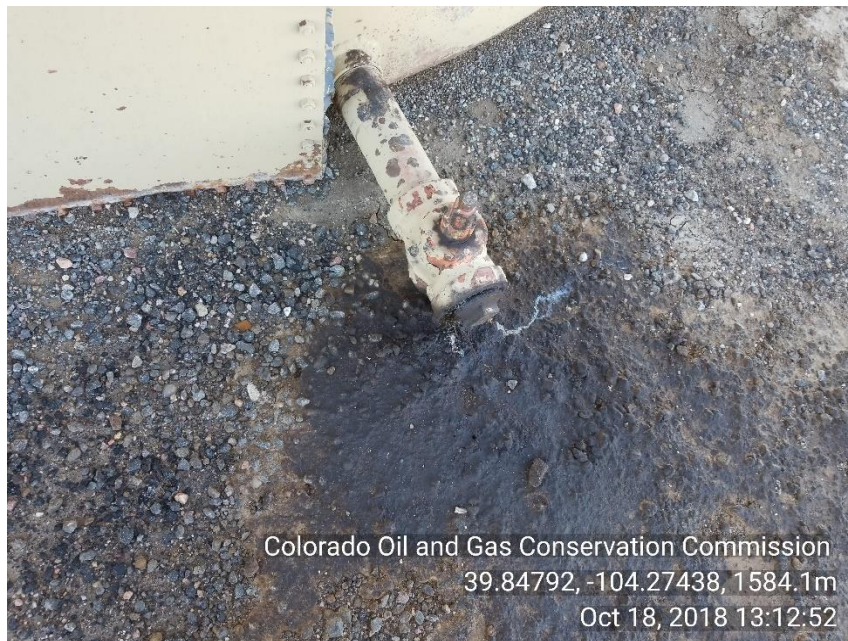
Photo 3 stained soil crude oil tank
