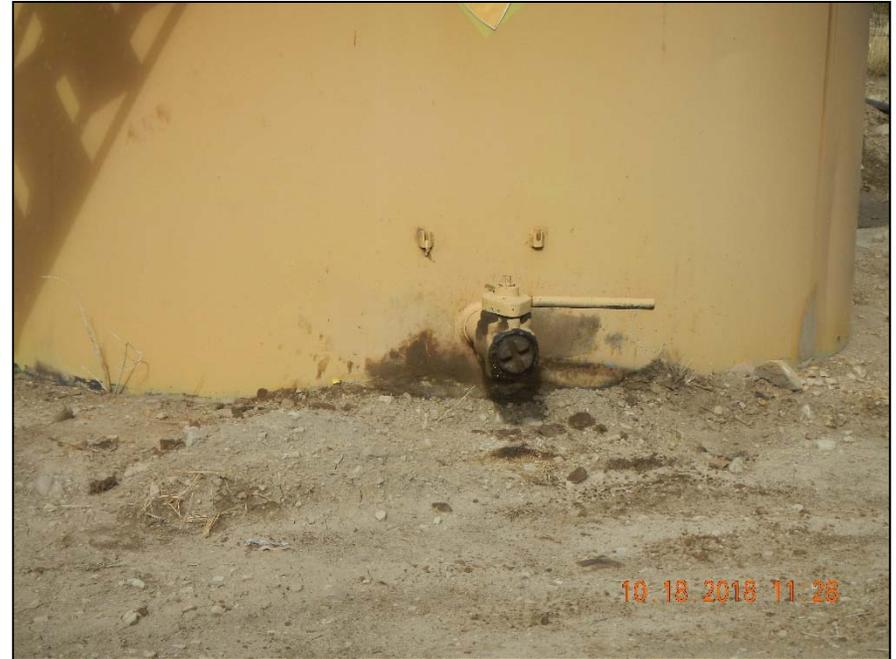
Photo 2. Stained soil at loadout.
