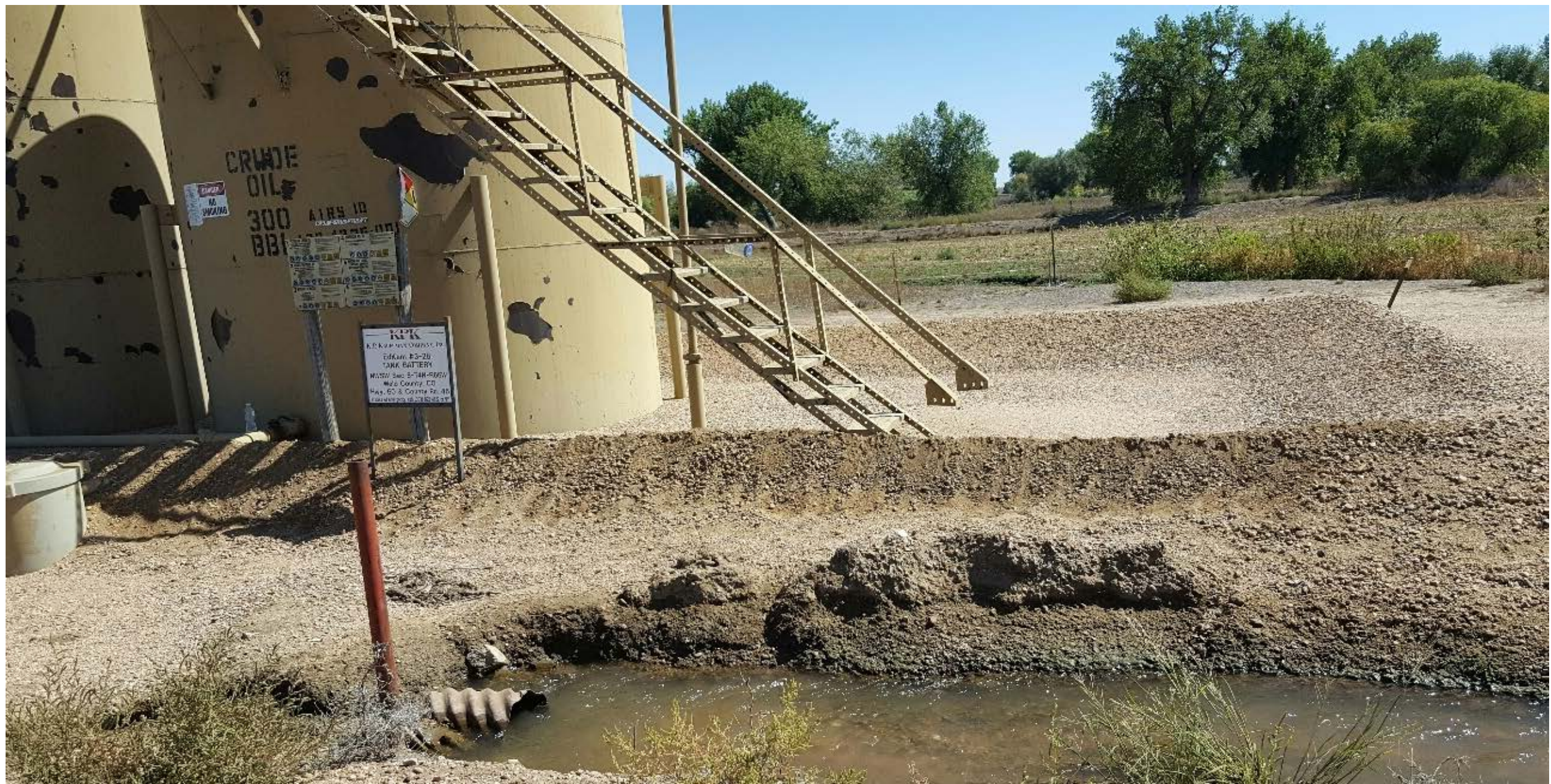
Figure #3 Berms around crude oil tank have been repaired.
