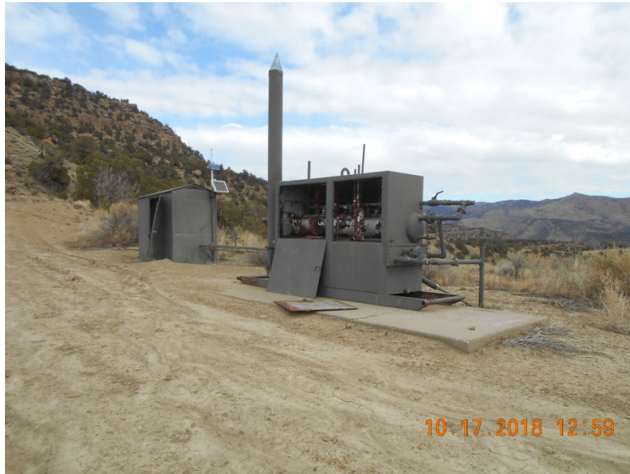
Separator and Meter housing
