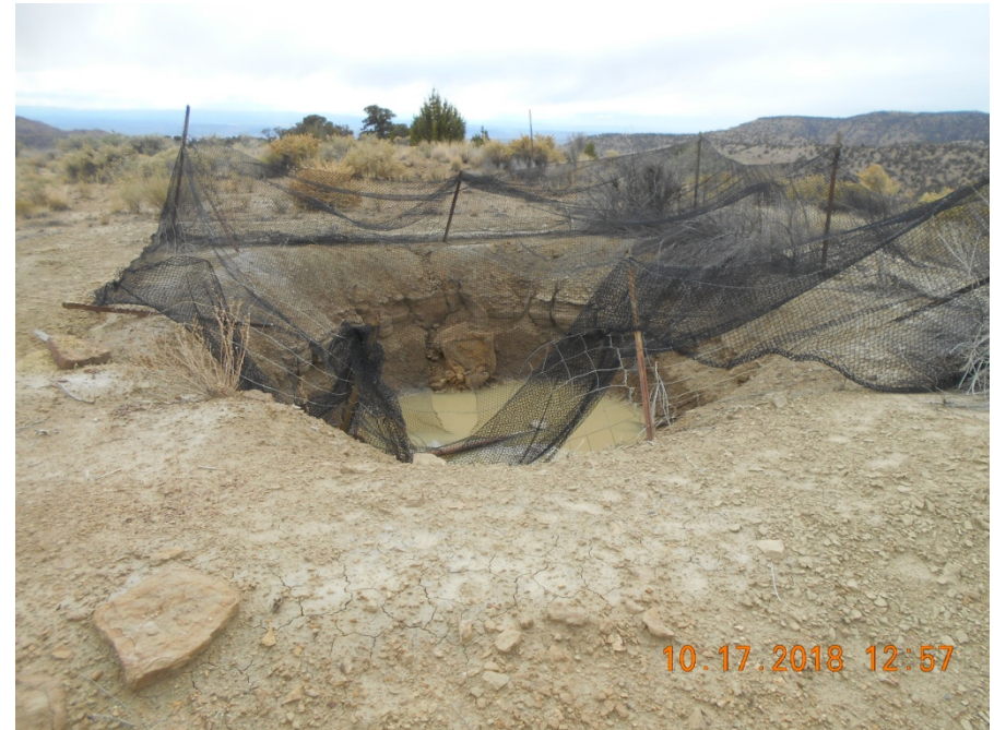
Blowdown pit with fencing and netting needs maintained.
