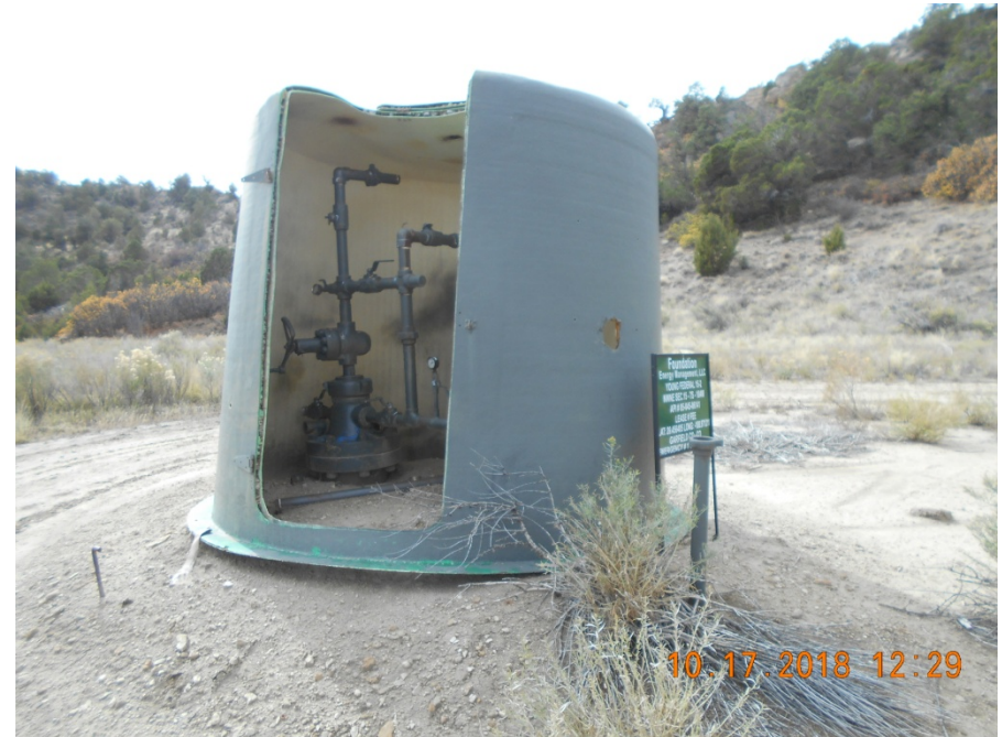
Wellhead inside housing
