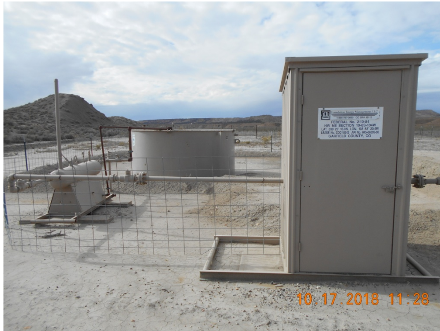
Separator, Meter housing and blowdown tank with fencing and sign
