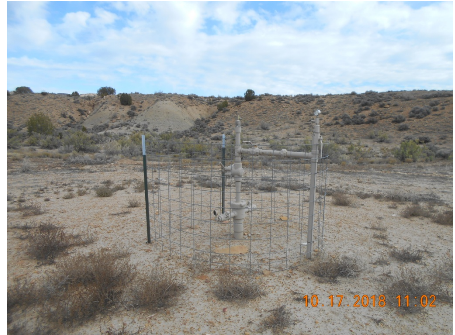
Wellhead with fencing
