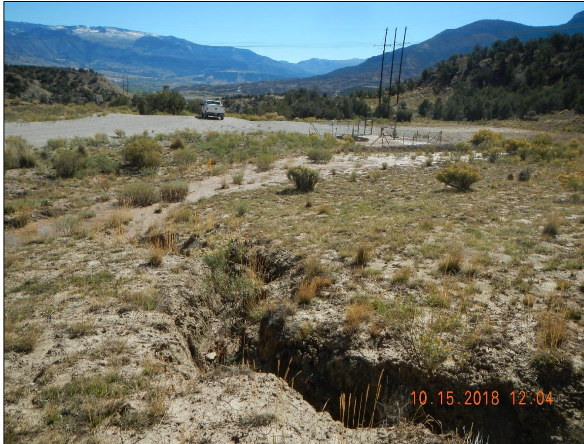
Deep erosion on drainage ditch.
