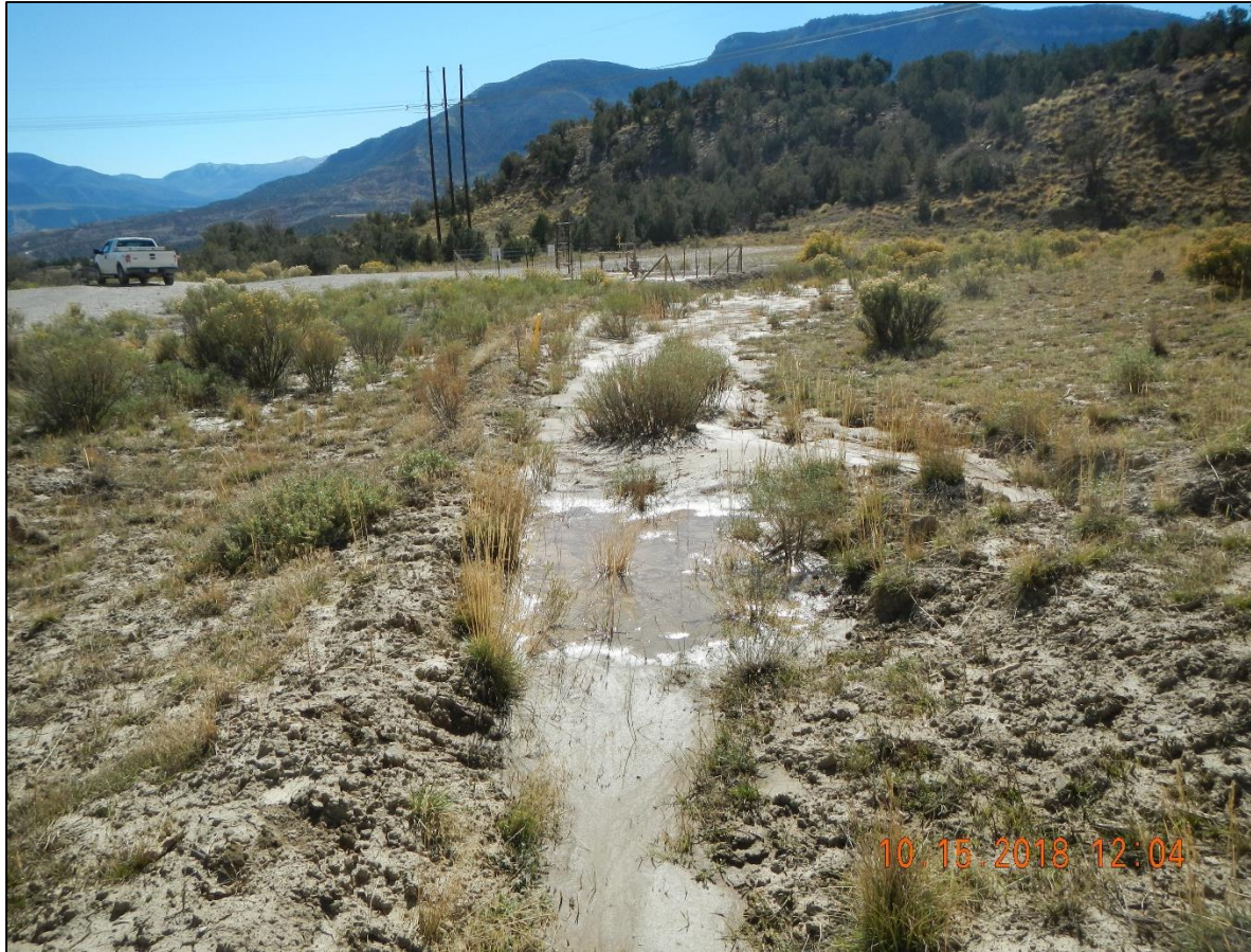
Sediment build up in ditch.
