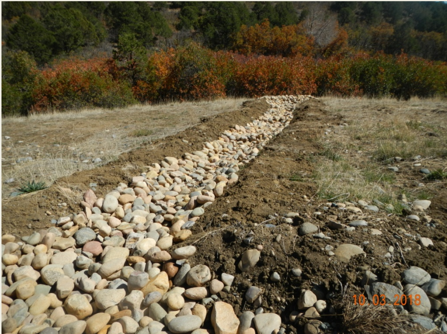
Photo 5. View of cobble run-down and silt trap within the eastern project area.
