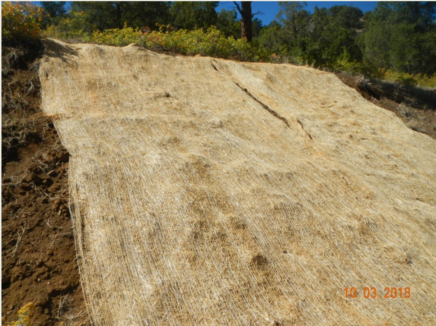
Photo 4. View of area in the western cut-slope where straw blanket was recently installed for erosion control.
