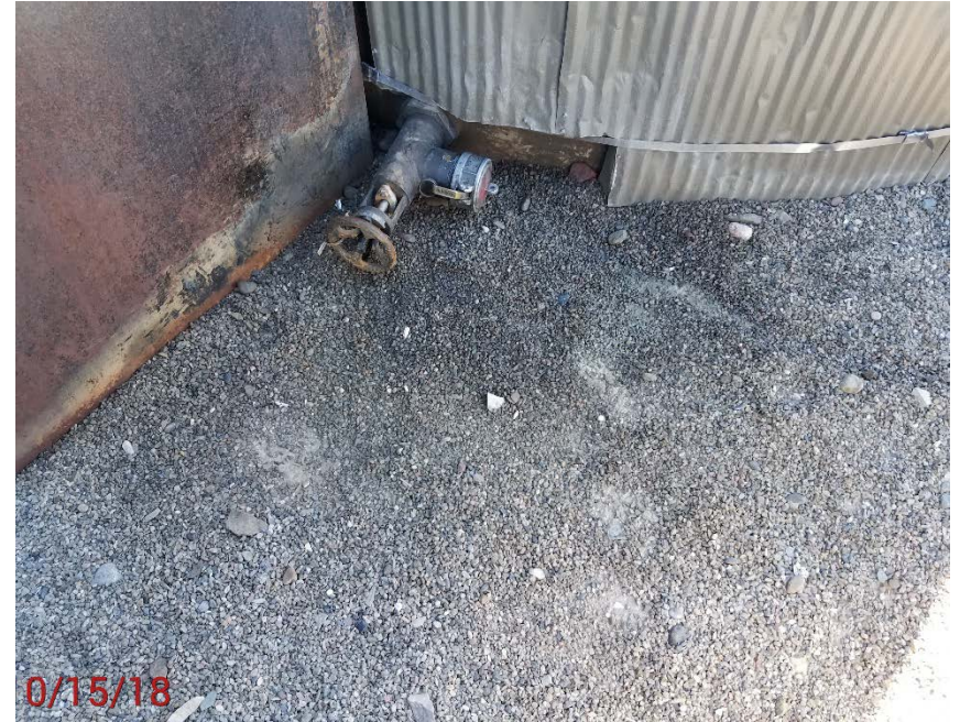
Location Photo #8, oily stained rock in battery containment
