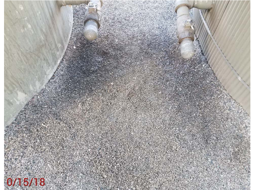
Location Photo #6, oily stained rock in battery containment
