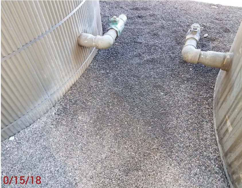
Location Photo #7, oily stained rock in battery containment
