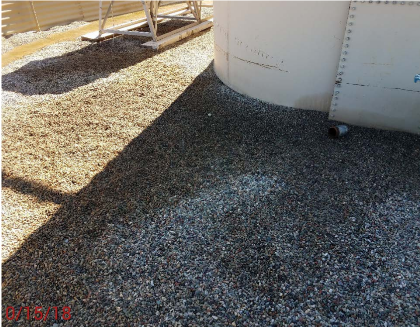
Location Photo #5, Stained rock in battery containment
