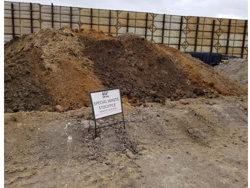
Photo #10 – Special Waste stockpile located east of SE cuttings stockpile. Hydrocarbon odor detected from stockpiled material on inspection date. Note that this stockpile has earthen berm on three sides.
