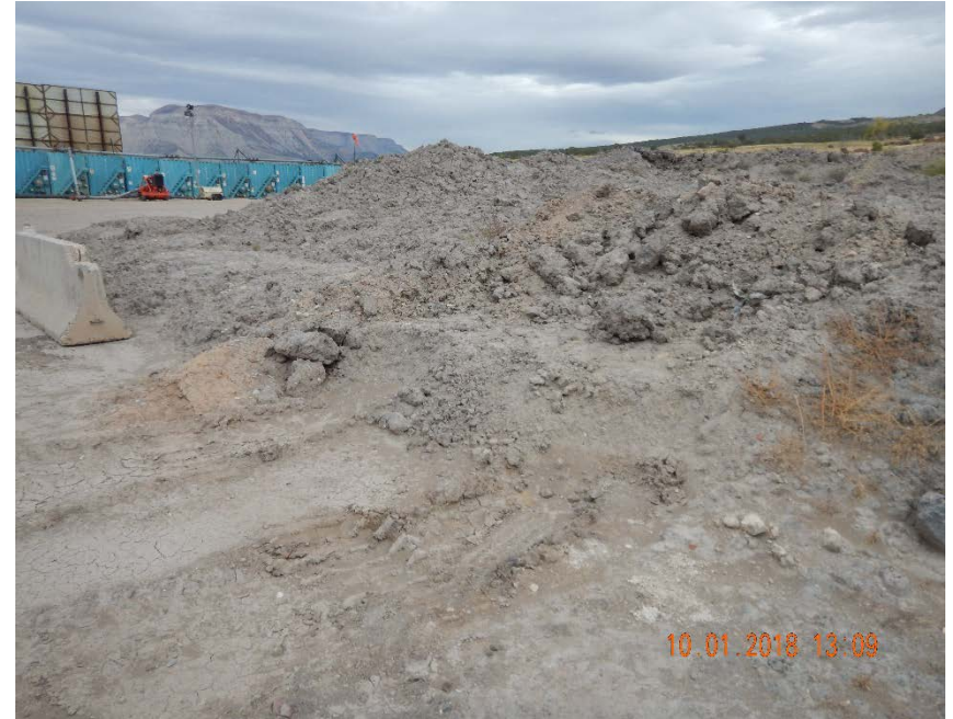
Photo #8 – Vegetation growth and lack of stormwater control at SE cuttings stockpile.
