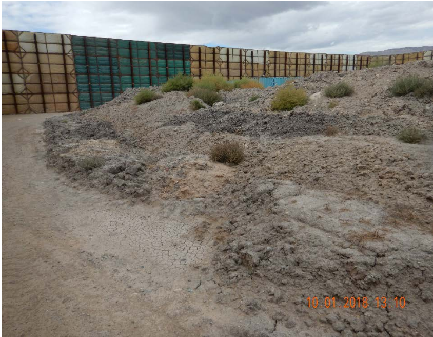
Photo #5 – Vegetation growth and lack of stormwater control at SW cuttings stockpile.
