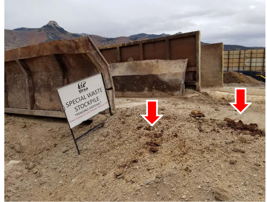
Photo #12 – Special Waste stockpile sign located in NE corner of pad outside of metal container. Note localized accumulations of oil-stained soil on ramp leading into container (red arrows).
