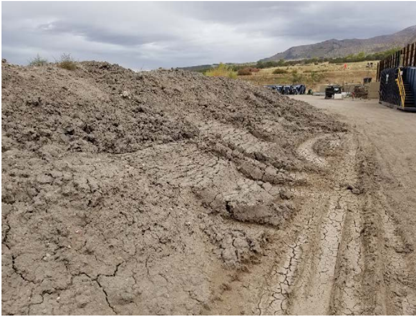
Photo #9 – View along south side of SE cuttings stockpile. Note lack of stormwater control and presence of tire tracks along stockpile.
