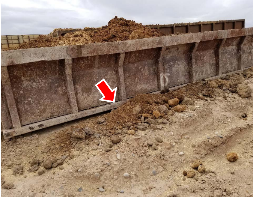
Photo #13 – View of NE Special Waste stockpile from north side. Hydrocarbon odor detected from stockpiled material on inspection date. Note stockpiled material accumulation outside of metal container (red arrow). Operator was instructed to remove this impacted material during inspection.
