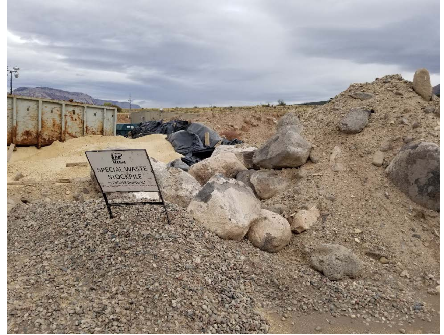
Photo #14 – Additional Special Waste stockpile located in NE corner of pad did not appear to contain hydrocarbon-impacted material. Note presence of soil, boulders, road base, sawdust, wooden debris, black plastic, and vegetation. Pile also lacks stormwater control.
