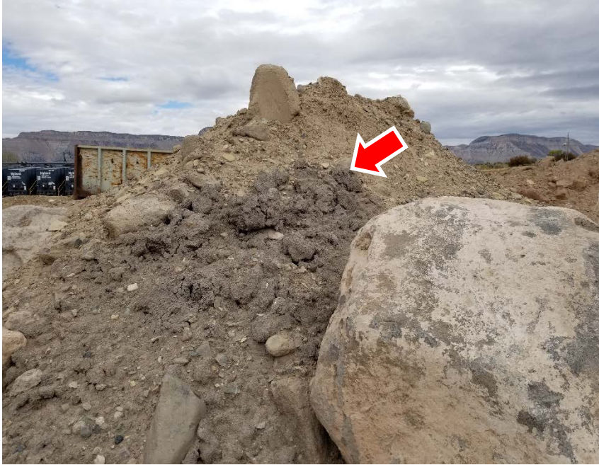
Photo #15 – Cuttings were also present in NE Special Waste stockpile (red arrow).
