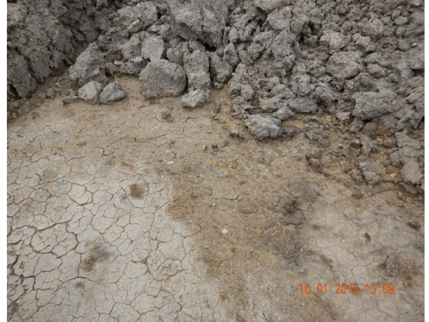
Photo #4 – Evidence of stormwater runoff and sediment transport at SE corner of cuttings stockpile.
