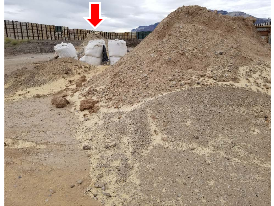
Photo #16 – View of NE Special Waste stockpile from the east. Note white materials storage containers within stockpile (red arrow) and absence of stormwater control on this side of stockpile.
