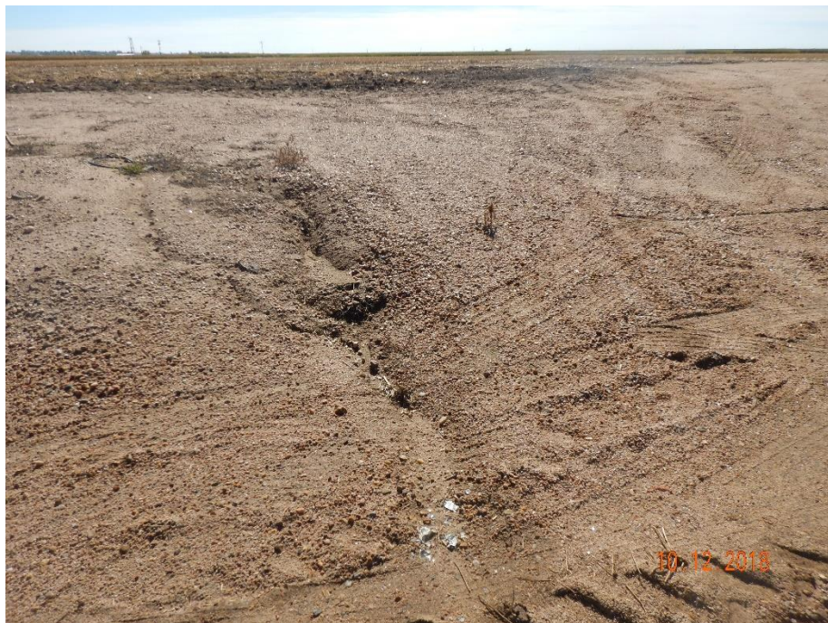
Photo 3: Photo taken from the north end of the location, facing south. Photo shows erosion degradation due to stormwater runoff from the pad. Erosion will need to be repaired, pad will need to be stabilized and BMPs implemented.
