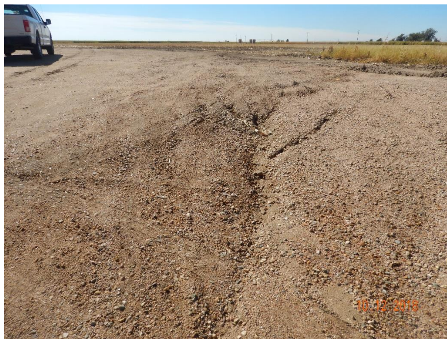
Photo 4: Photo taken from the north end of the location, facing south. Photo shows erosion degradation due to stormwater runoff from the pad. Erosion will need to be repaired, pad will need to be stabilized and BMPs implemented.
