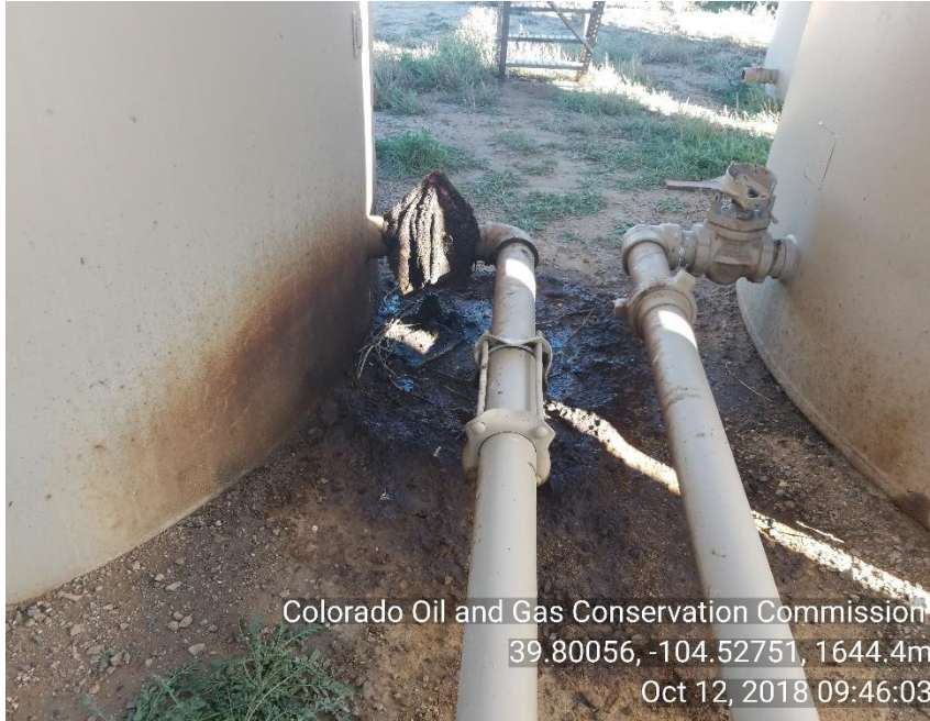
Photo 1 stained soil between crude oil tanks
