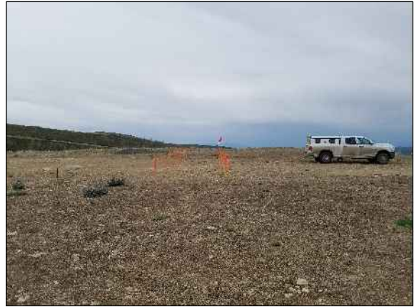
WELL LOCATION LOOKING SOUTH 8/3/2017
