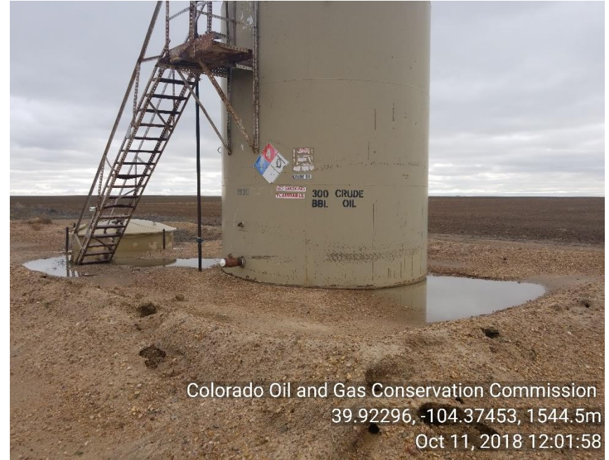
Photo 2 TNK BTRY Berm cannot hold volume of tank's
