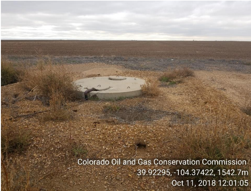
Photo 35 Produced water tank no signage
