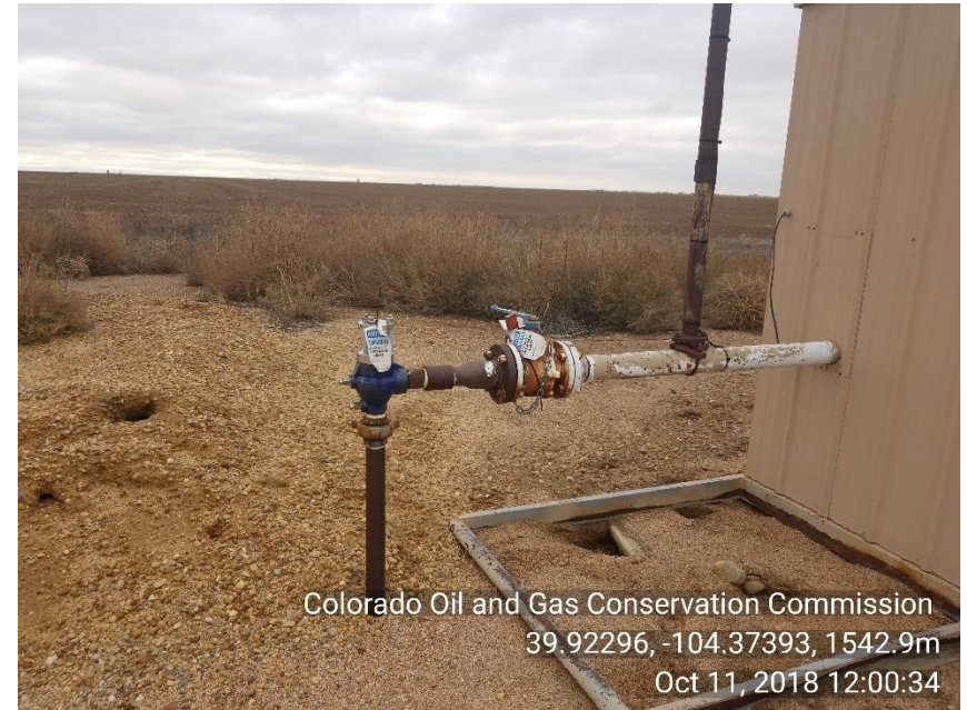
Photo 4 Meter house locked out tagged out
