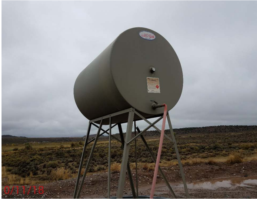
Location Photo #3, missing sign
