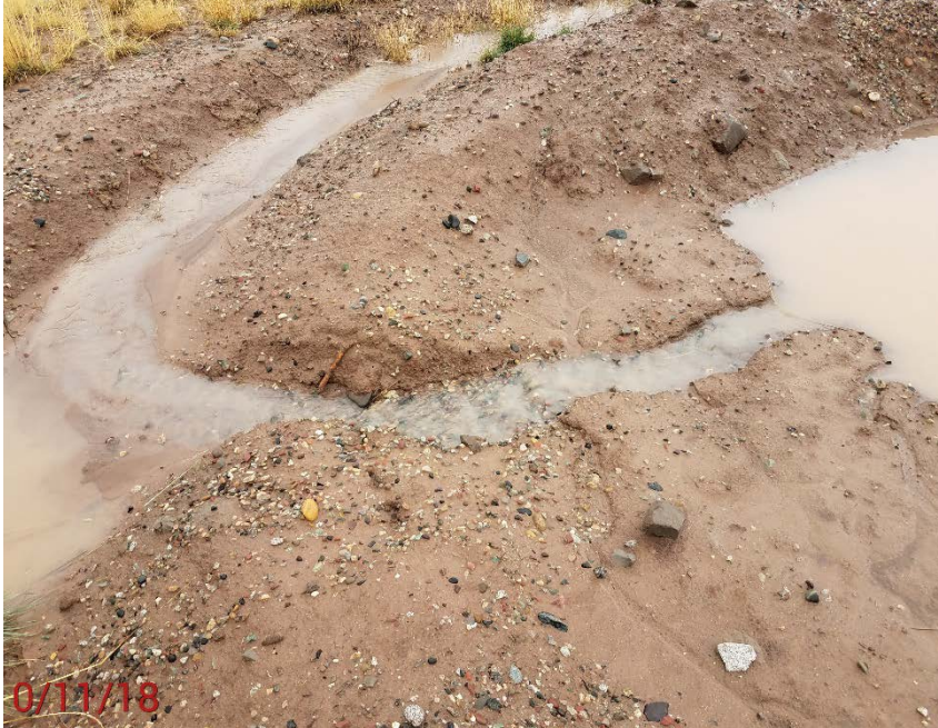
Location Photo #13, storm water issue, sediment being moved off location.
