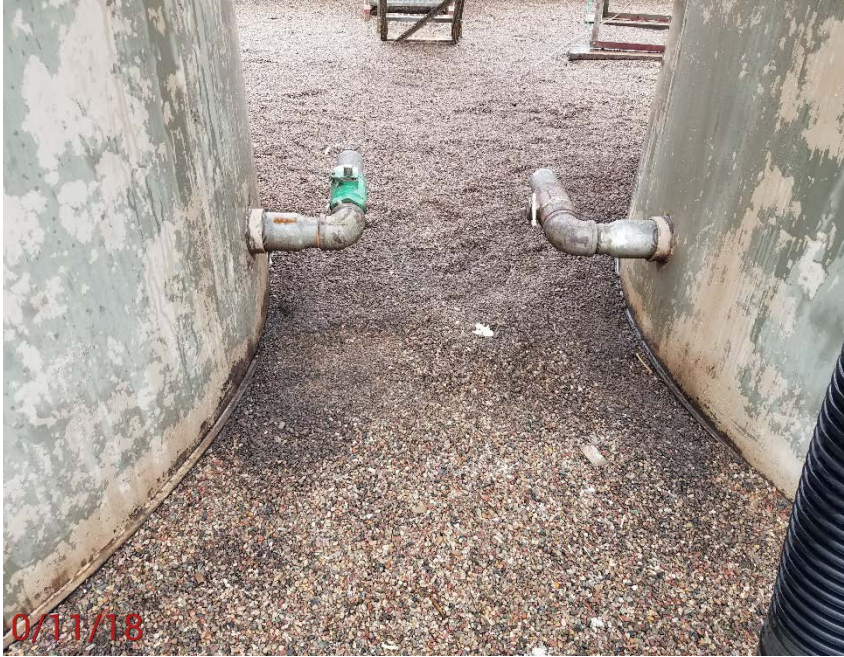
Location Photo #9, stained rock in battery containment.
