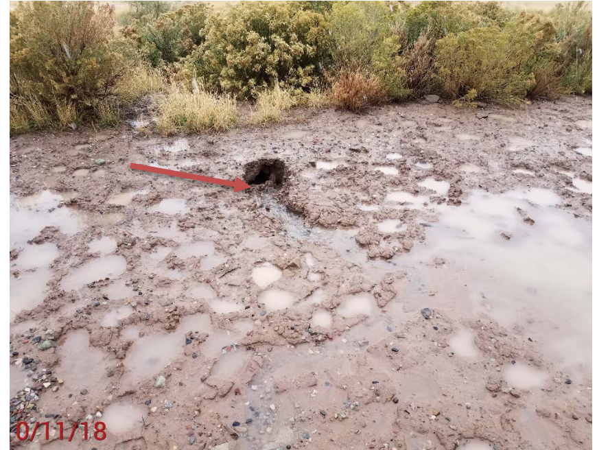
Location Photo #6, hole in berm, south corner of separators.
