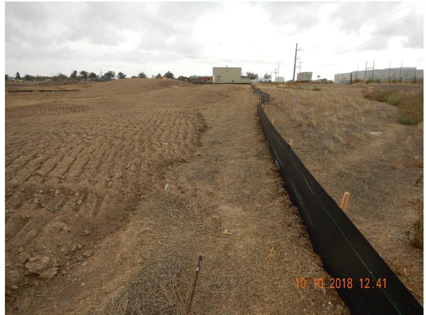
Photo 2. Photo taken from the western perimeter of the location, facing South. Silt fence BMP has been installed around the perimeter of the location.
