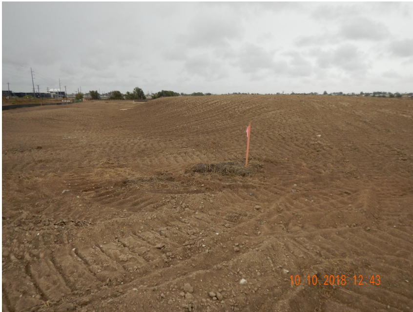
Photo 3. Photo taken from the southwestern perimeter of the location, facing North. Photo illustrates the topsoil stockpile stored along the southwestern perimeter of the location. Topsoil has been temporarily stabilized with equipment tracking.
