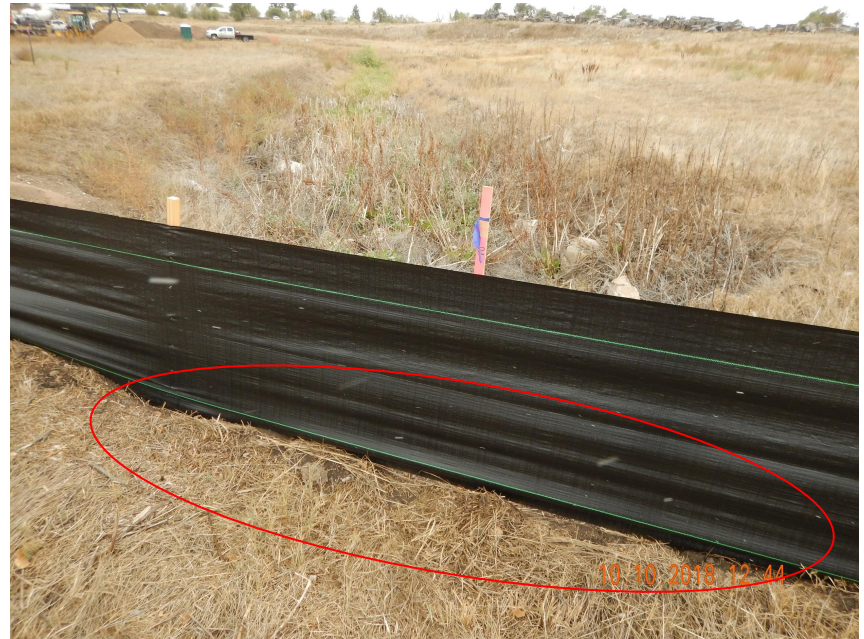
Photo 4. Photo taken from the southern perimeter of the location, facing South. Photo illustrates a portion of the silt fence that has not been properly trenched.
