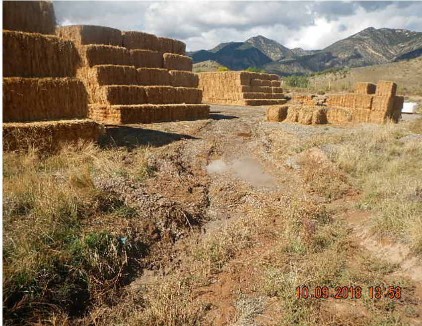
Drain path moving off of pad, no stabilization or BMP's
