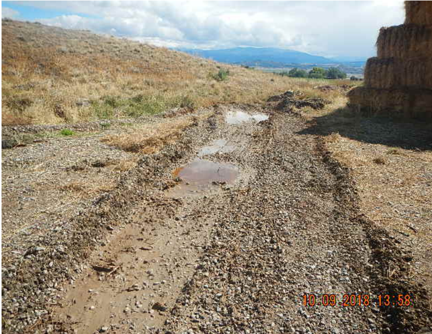
Drain path cut into pad to move storm water away from hay
