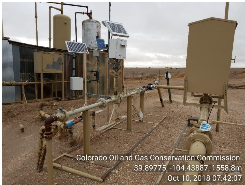
Photo 5 Gas meter run all vlv's locked out tagged out
