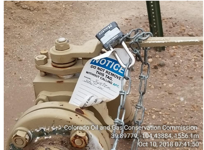
Photo 4 Sales line Locked out tagged out
