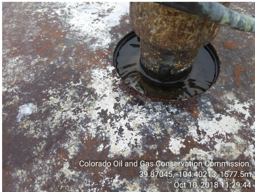
Photo 3 WH leaking around top plate of WH
