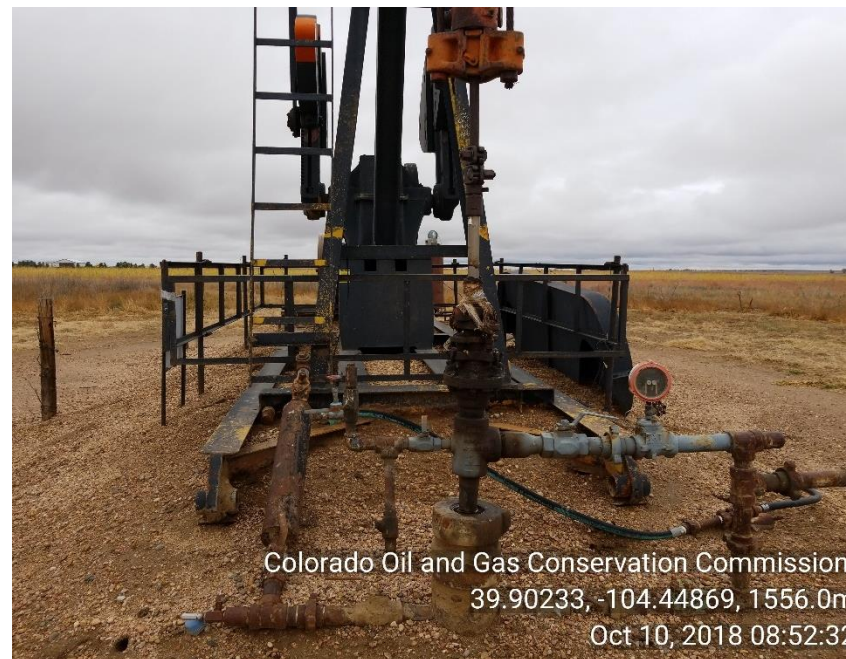
Photo 2 rags and tape around polish rod and packing
