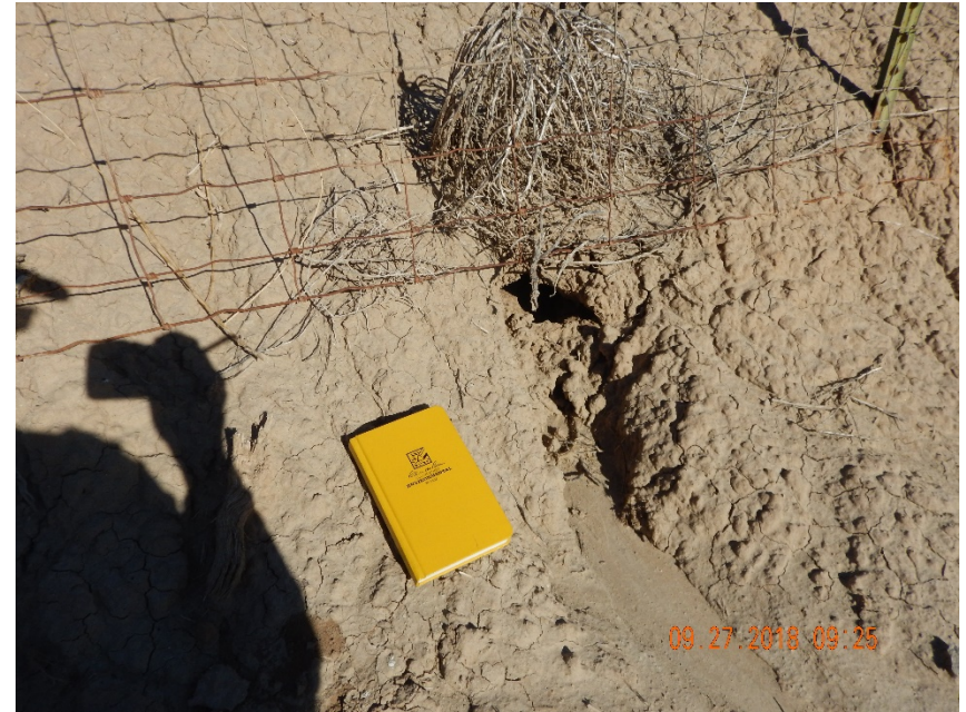
Photo #10 –Evidence of erosion (and apparent subsurface soil piping) observed in east pit berm.
