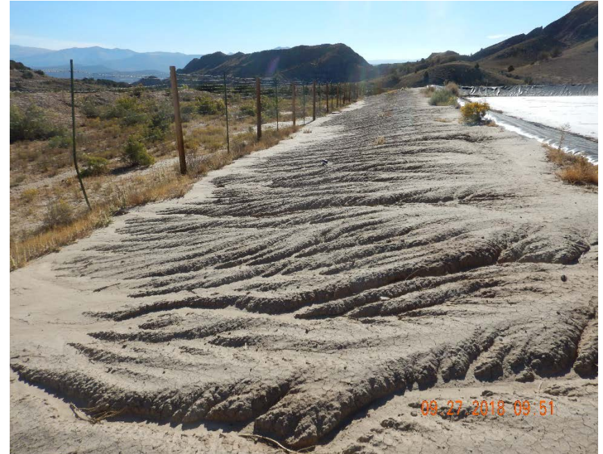
Photo #20 – Erosion rills along north pit berm resulting in off-site sediment transport north of pit.
