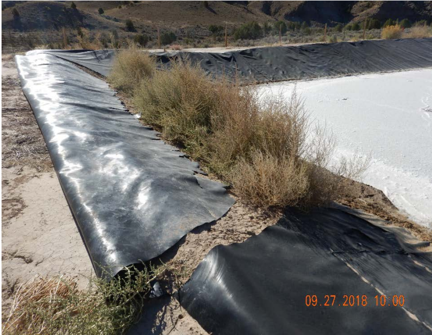
Photo #23 – Approximately 30’ section of pit liner has been completely separated from pit and was rolled back into place without being sealed or repaired. Note that area of berm formerly underlying pit liner now supports vegetation.
