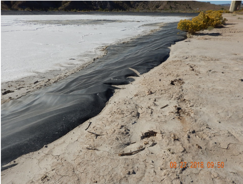
Photo #19 – Evidence of sediment transport into pit and mud cracks resulting from apparent pooling of storm water in shallow area at NW corner of pit berm.
