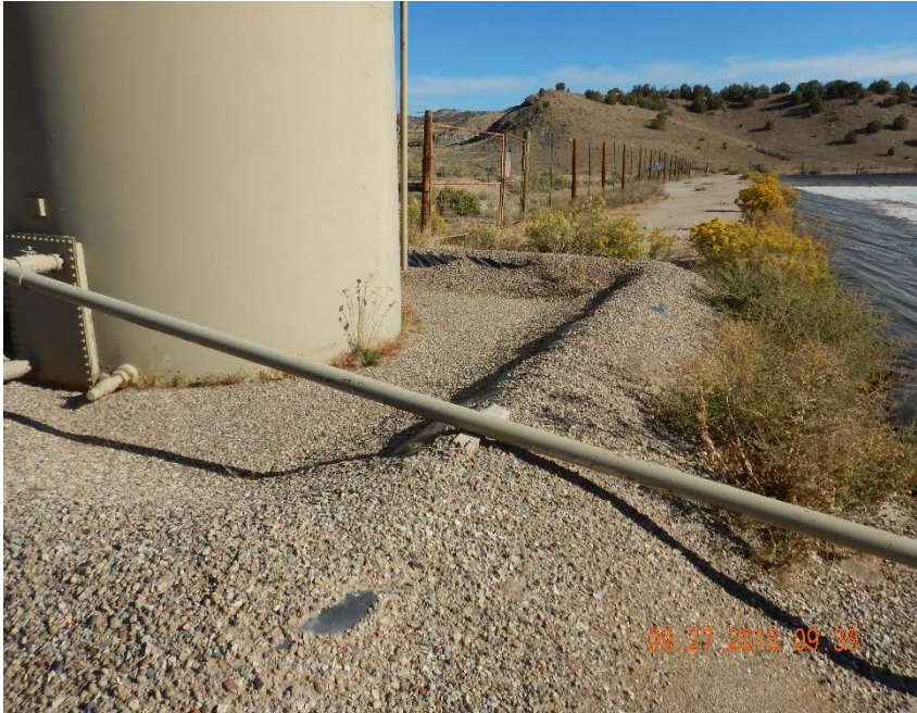
Photo #17 –Vegetation growth along anchor trench, pictured on west side of pit, was present along all sides of pit on inspection date.
