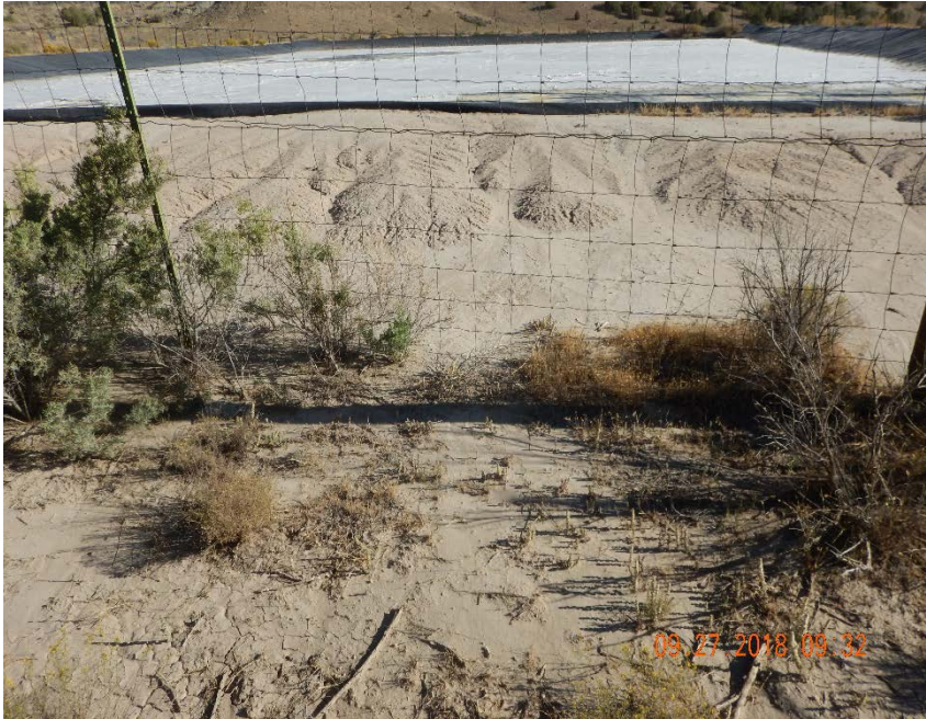
Photo #13 – Erosion and off-site sediment transport from south pit berm.
