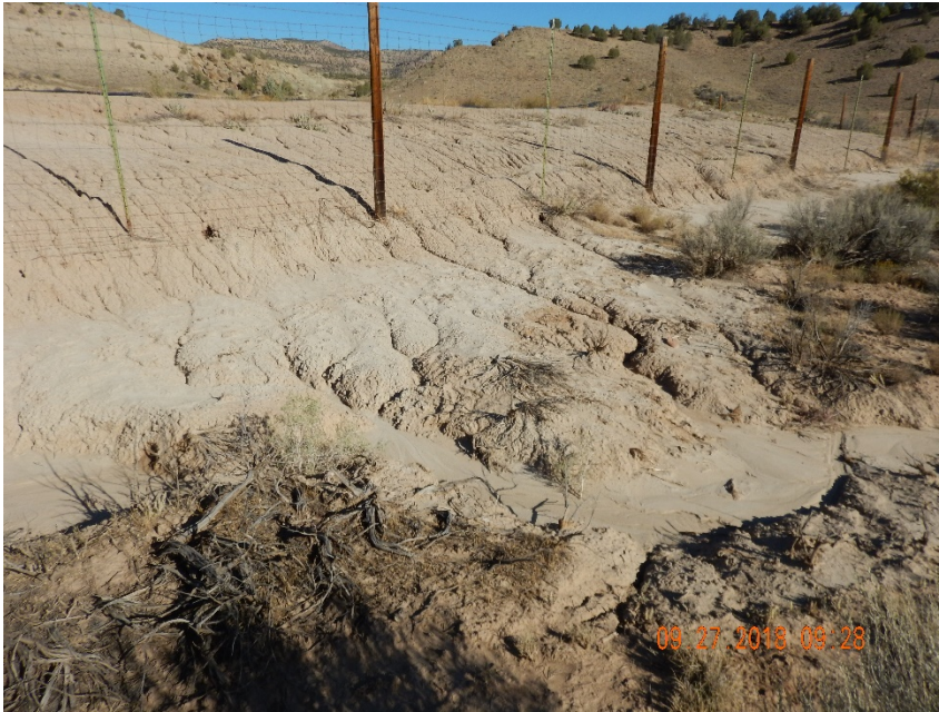
Photo #11 – Berm erosion and off-site sediment transport to east of pit. Stormwater and sediment flow toward mapped surface water feature, Coon Hollow, located approximately 200' east of pit.
