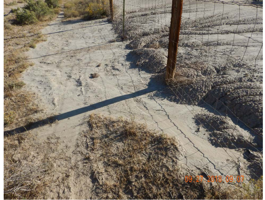
Photo #6 – Erosion of western pit berm and off-site sediment transport into stormwater channel.
