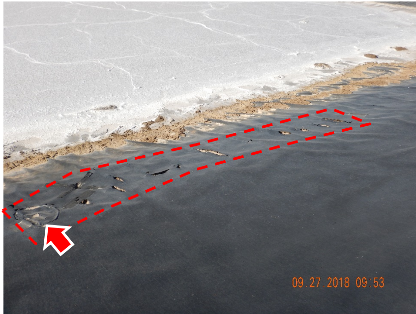
Photo #21 – Examples of holes observed in pit liner (outlined in red), primarily along north side of pit. Over sixty (60) holes were observed in visible portion of pit liner on inspection date, some of which had been previously patched by operator (red arrow).
