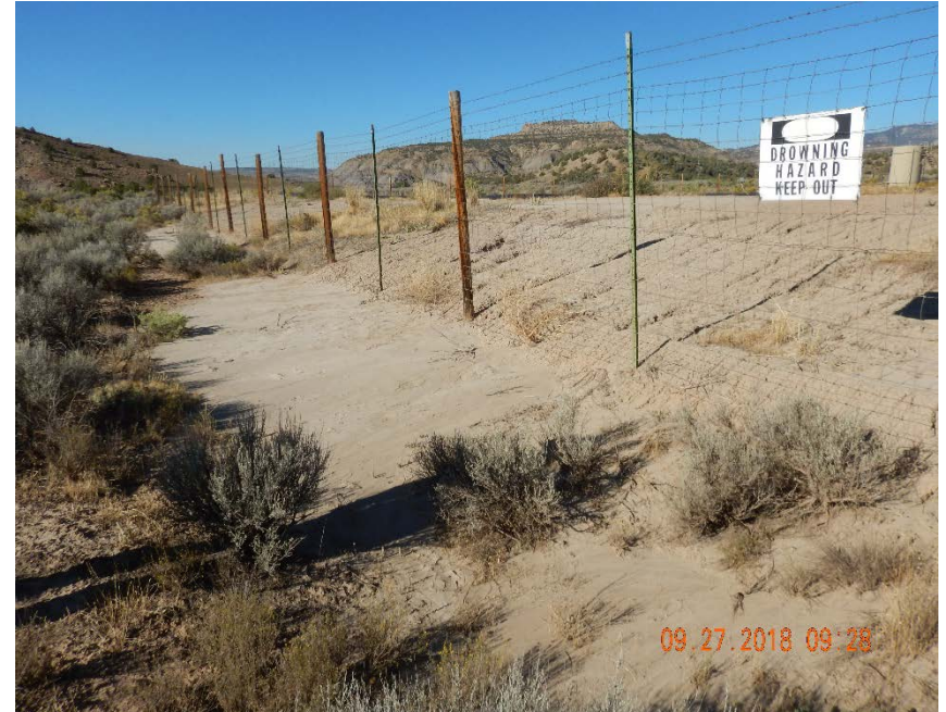
Photo #12 – Additional erosion and off-site sediment transport from east pit berm.
