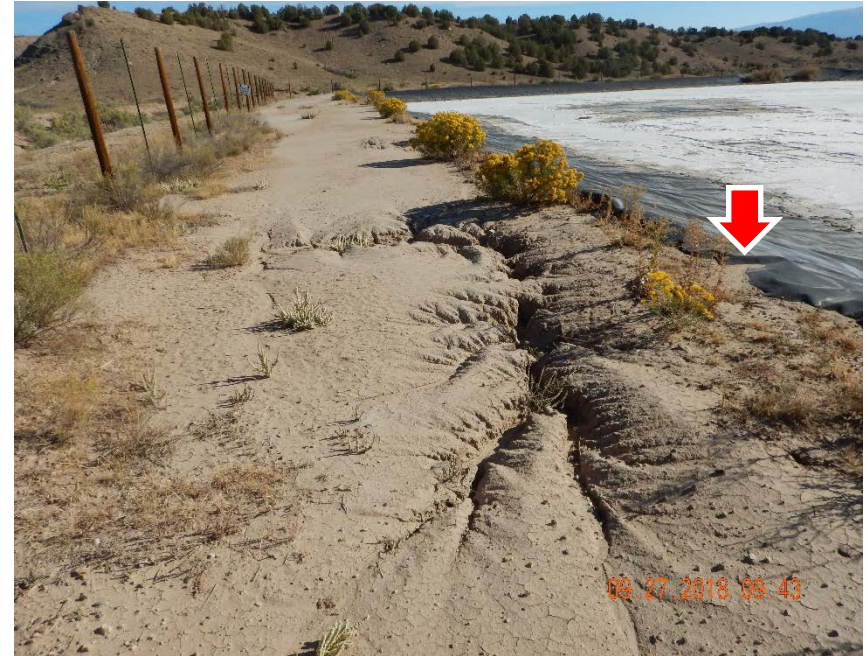
Photo #18 – Erosion rill on west pit berm resulting from apparent subsurface soil piping and stormwater flow. Note evidence of sediment transport into pit (red arrow).
