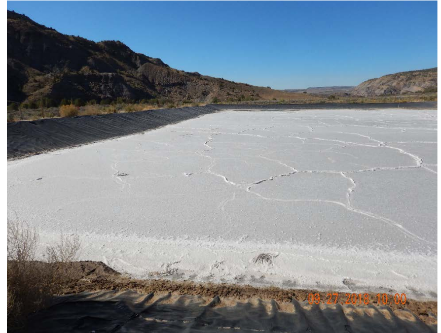
Photo #24 – View of salt and sediment covering lined pit bottom. Liner beneath salt and sediment could not be visibly inspected for integrity issues. Liner integrity issues along pit bottom have been documented under Remediation Project #8494 and Spill/Release ID #443917.
