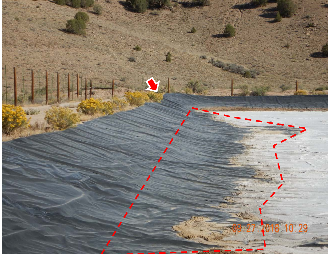
Photo #29 – View along west pit berm from SW corner of pit illustrates: 1) low area in NW corner of pit berm (red arrow) and 2) irregular surface along base of pit berm resulting from apparent sediment transport beneath pit liner (outlined in red).
