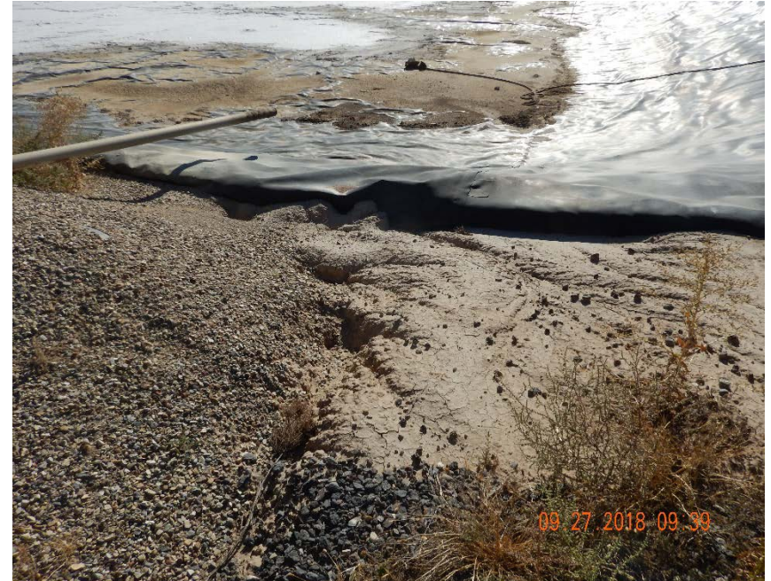
Photo #16 – Evidence of berm erosion, stormwater flow into anchor trench/beneath liner located at SW corner of pit near inlet from produced water tank.
