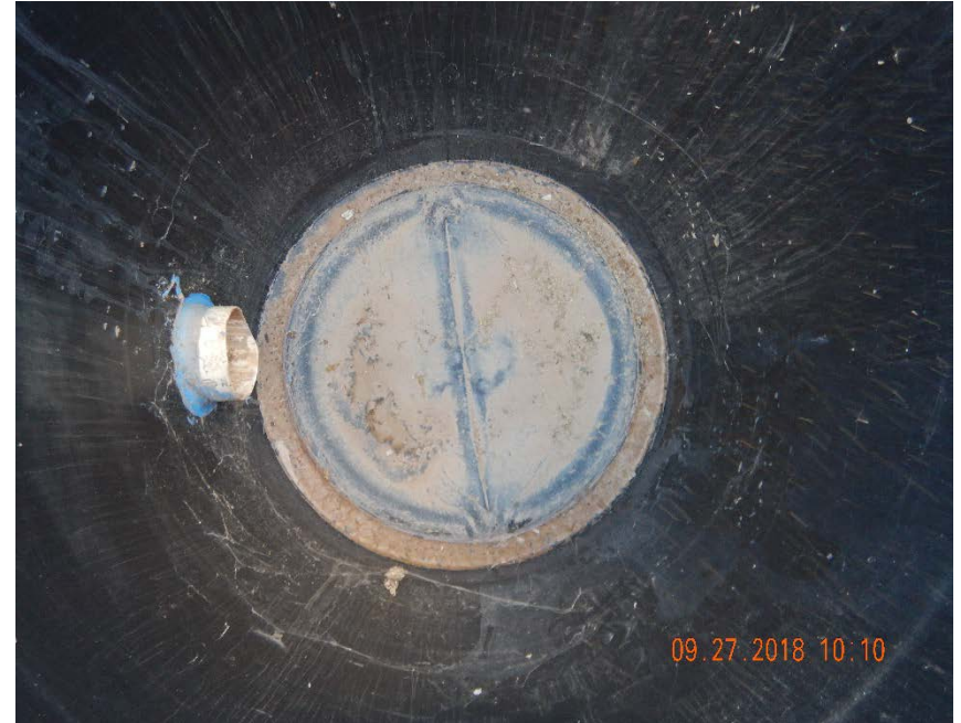
Photo #26 – Leak detection system was dry on date of inspection.
