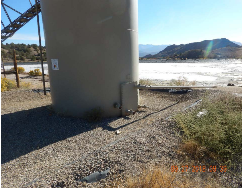
Photo #15 – Tank berm at SW corner of pit is shallow and eroded. Note produced water tank lacked truck loadout assembly on inspection date.
