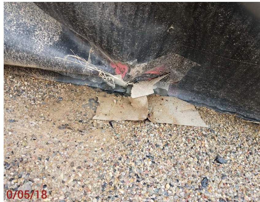
Location Photo #4, hole in secondary containment liner
