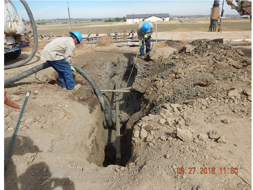
Hydro – excavation work being completed to expose flowlines in the area of release (view North)
