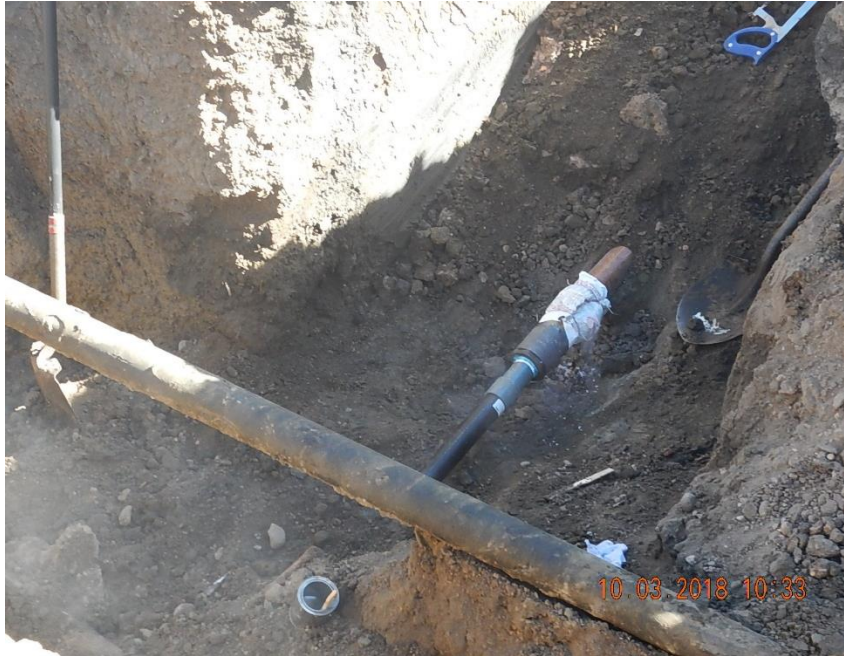
Repairs/ replacement section of flowline (2" HDPE) being installed/ connected to the existing flowline pipe on the south end of the excavation.
