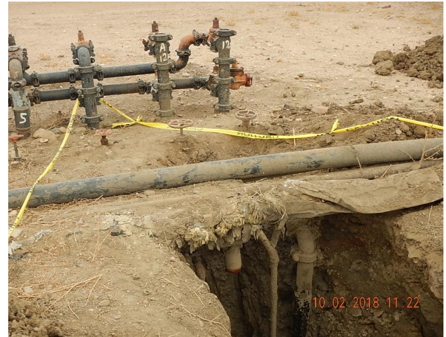
An external corrosion hole was found on the 3" un-coated carbon steel flowline associated with the Amoco-Charter-Schneider 12A well (API 123-09038); a section of this flowline was removed.
