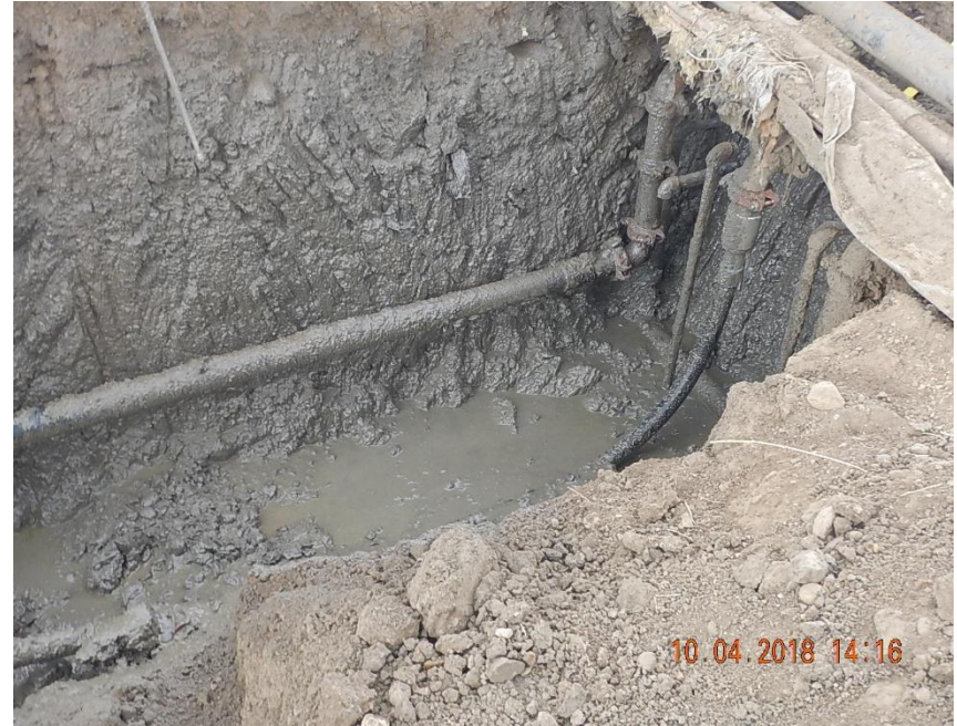
Replacement section of flowline connected to the flowline manifold on the north end of the excavation.
