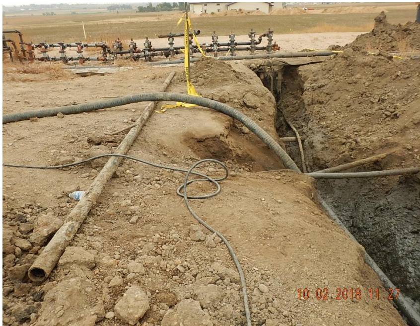
Approximately 20' of 3" flowline was cut out and removed from the excavation (shown on left side of photo)
