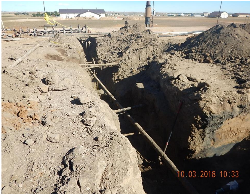
Excavation work exposed numerous flowlines in the area of release south of the flowline manifold (pictured at top).
