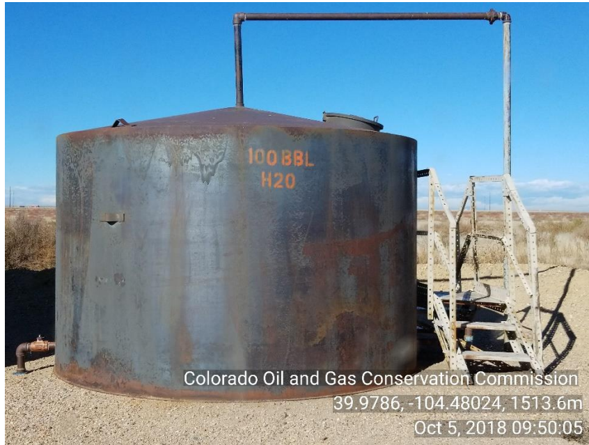
Photo 3 Produced water tank
