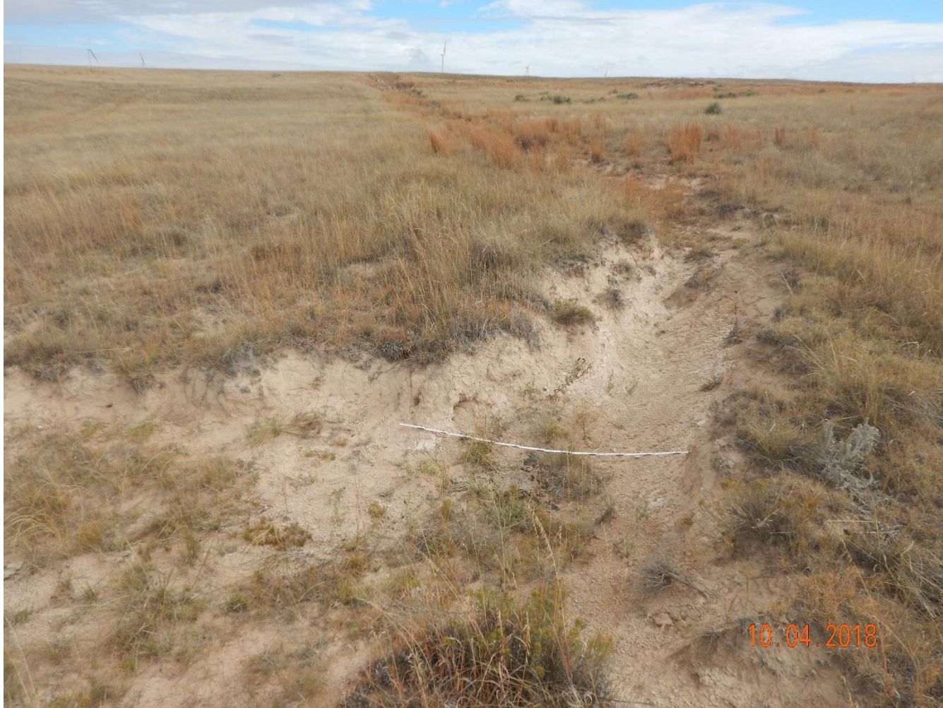
Photo 5: Photo taken from the east end of the location, facing northeast. Photo shows gully erosion. Photo also shows access road has not been recontoured/regraded to that of the adjacent lands, and stormwater has continued to degrade and channelize the access road creating a gully. 6 foot measuring stick for reference.
