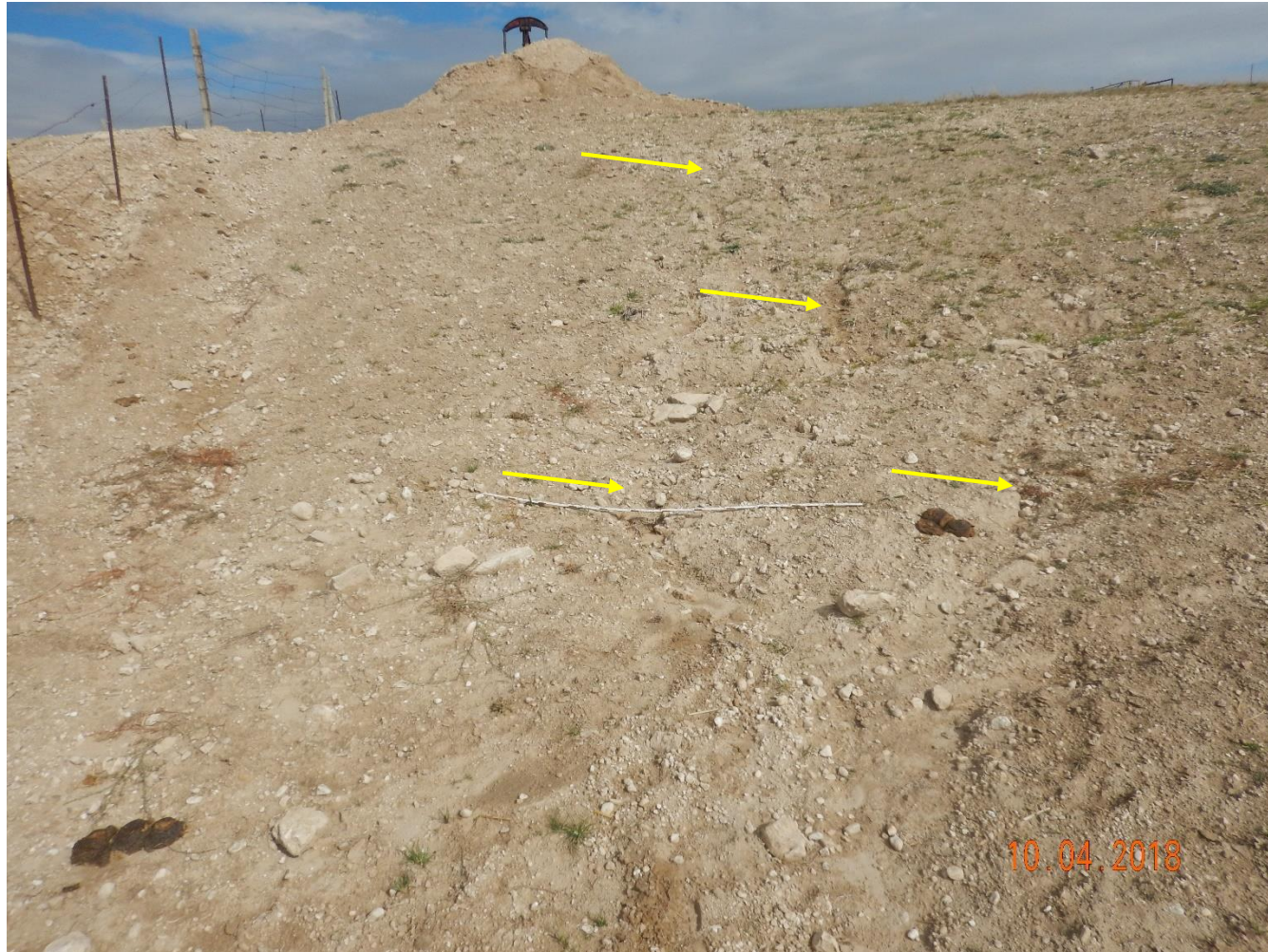
Photo 3: Photo taken from the southeast end of the pit, facing north towards the well. Photo shows areas of the interim that operator previously regraded and seeded. Operator failed to implement required stabilization or stormwater and erosion control BMPs per CAs. Photo shows erosion degradation has been allowed to continue. 6 foot measuring stick for reference
