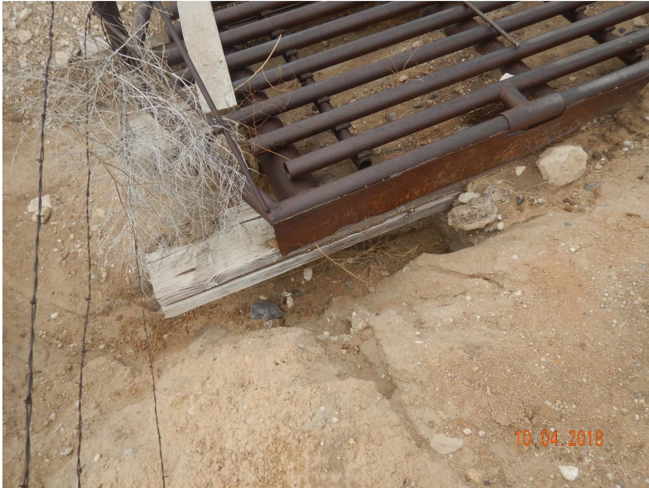
Photo 13: Photo taken from the cattle guard at the access road entrance. Photo shows erosion degradation has not been repaired; stormwater erosion has cut underneath the cattle guard.
