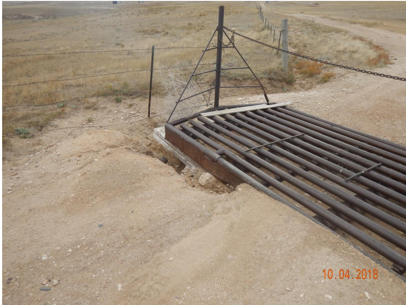
Photo 12: Photo taken from the cattle guard at the access road entrance. Photo shows erosion degradation has not been repaired; stormwater erosion has cut underneath the cattle guard.
