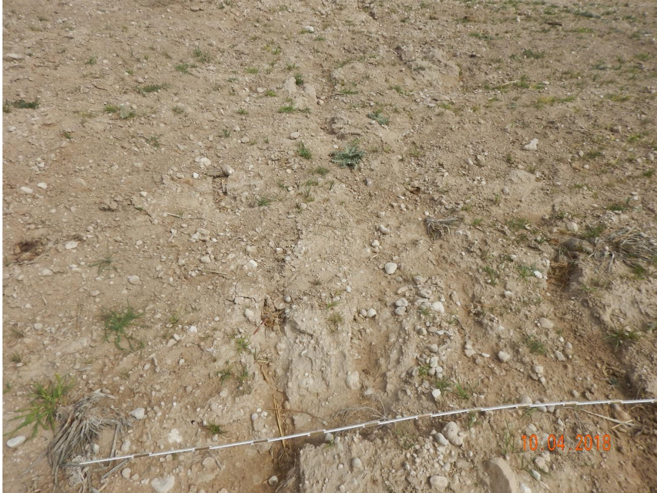
Photo 4: Photo taken from the southeast end of the pit, facing north towards the well. Photo shows areas of the interim that operator previously regraded and seeded. Photo shows Operator has failed to implement required stabilization, stormwater and erosion control BMPs per Cas; erosion degradation has been allowed to continue. 6 foot measuring stick for reference.
