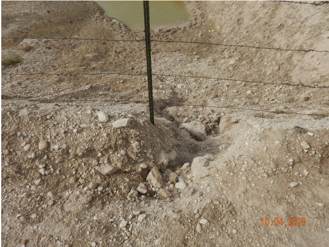
Photo 11: Photo taken from the east end of the pit, facing west. Photo shows erosion degradation (gully) has reformed. Production areas have not been sufficiently stabilized.
