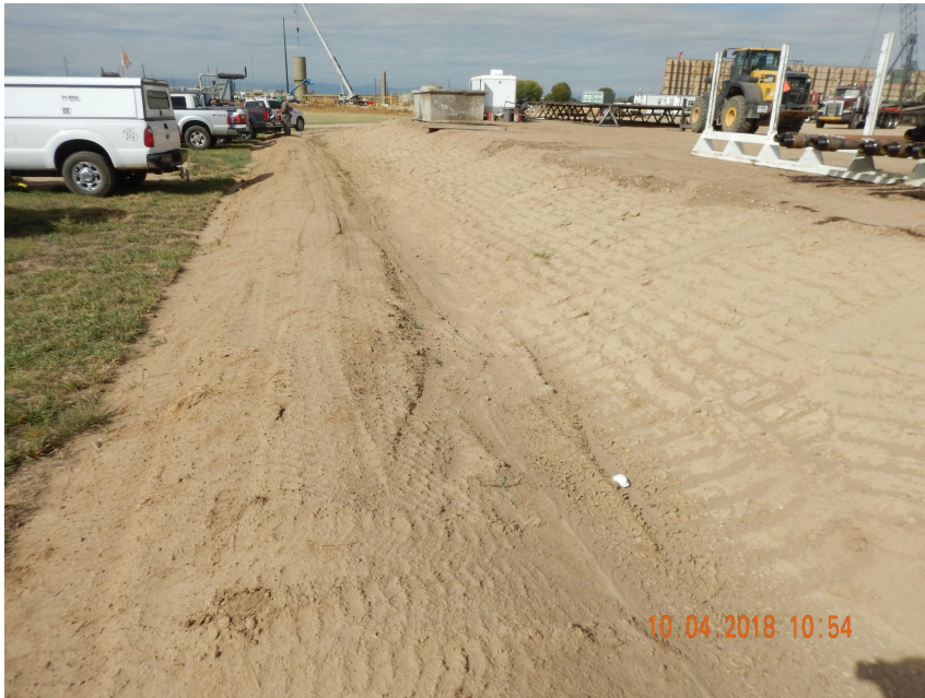
Photo 1. Photo taken from the southeast perimeter of the location, facing West. Ditch and berm BMP has been installed around the entire perimeter of the location. Rill erosion was observed along the southern, eastern and western fill slope areas, but did not discharge off location.
