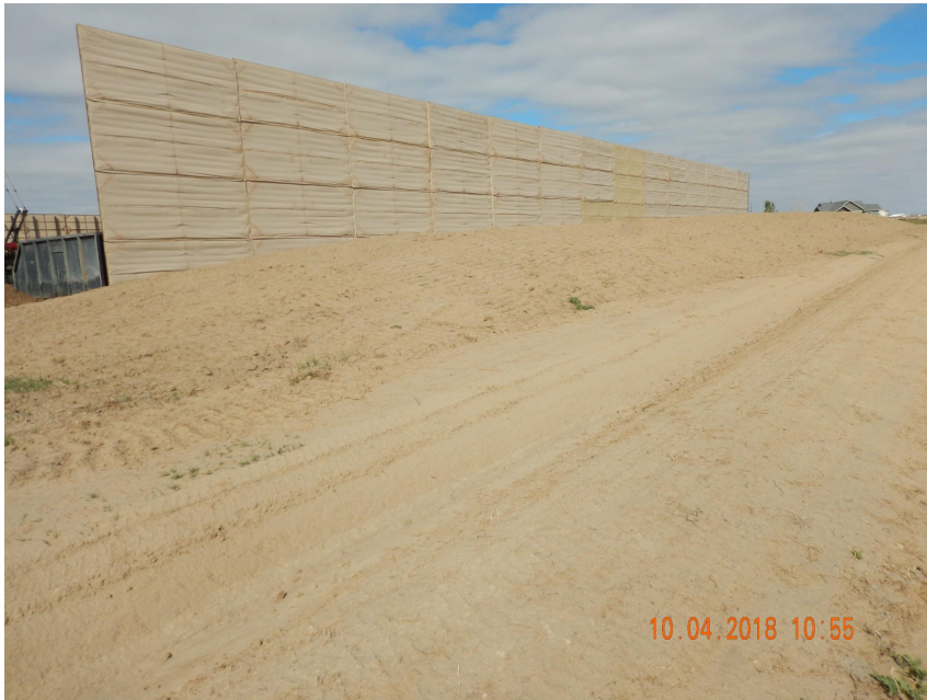
Photo 3. Photo taken from the eastern location, facing North. Operator has salvaged and stored topsoil along the eastern perimeter of the location. Topsoil has been temporarily stabilized with equipment tracking.
