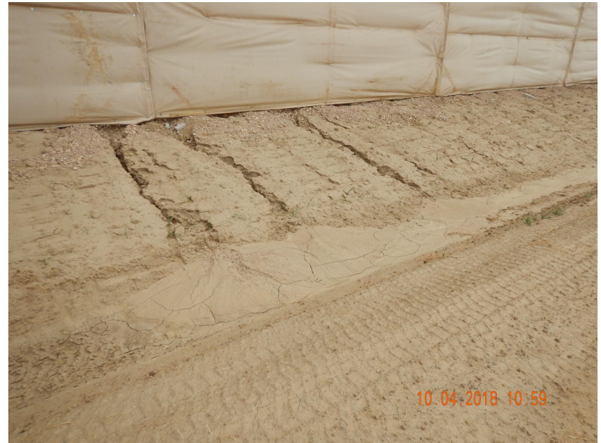
Photo 6. Photo taken from the western location. Photo illustrates rill erosion.
