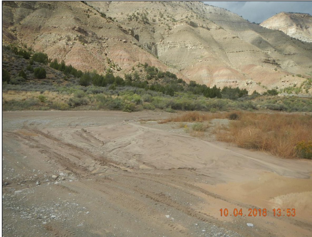
Sediment and water build up on main road and entrance road to MV 29-27 pad
