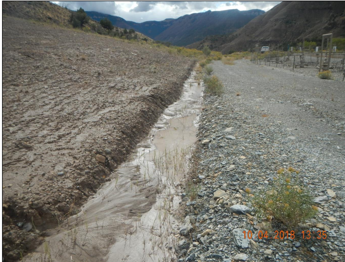
Sediment in ditch along cut slope.
