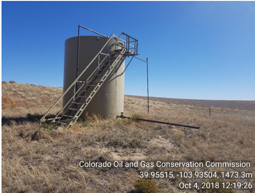
Photo 3 TNK BTRY no birm around tank, weeds around tank
