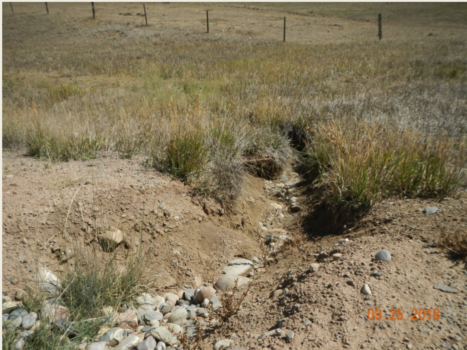
Photo 3. View of erosional channel in the eastern fill slope, appears to be partially stabilized with cobble. This needs to be monitored and additional erosion controls applied if it active erosion is occurring.
