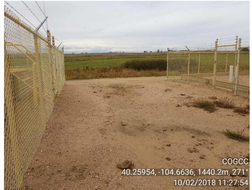
Photo 4– Erosion; sediment transported off west side of site
