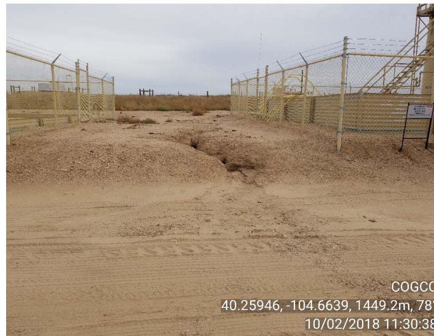
Photo 2 – Erosion; sediment transported off west side of site
