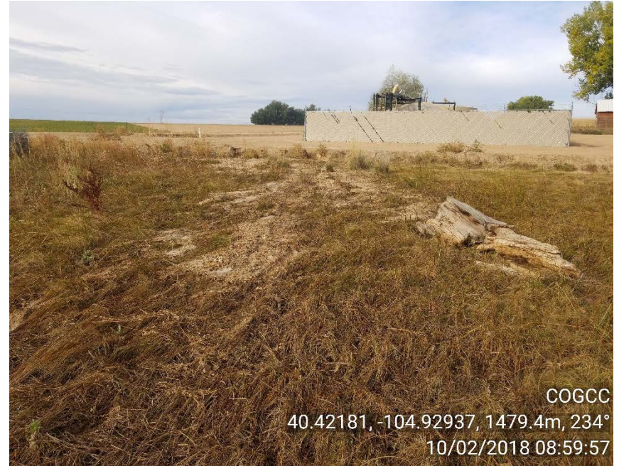
Photo 4– Erosion; sediment transported off east side of site
