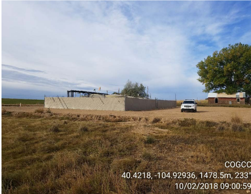
Photo 3 – Erosion; sediment transported off east side of site
