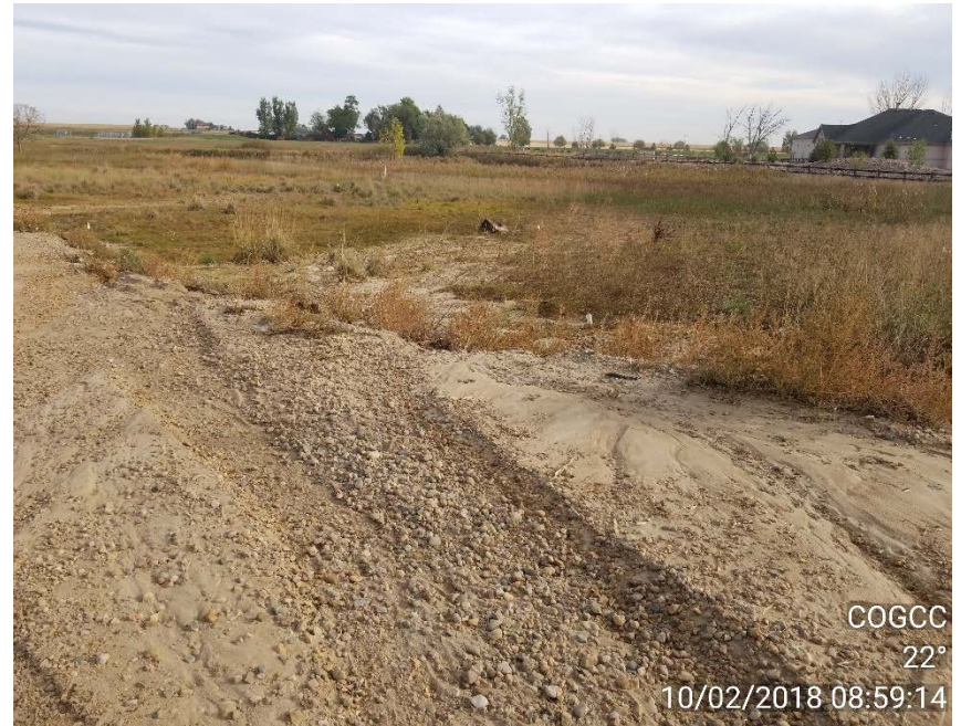
Photo 2 – Erosion; sediment transported off east side of site
