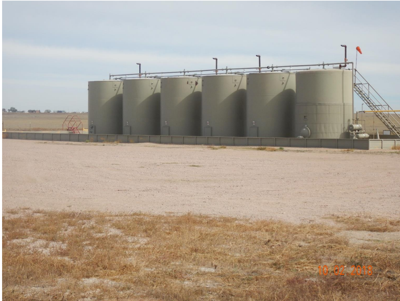
Photo 5: Photo of tank battery. 6 total 300 bbl AST; 5 crude, 1 produced water.
