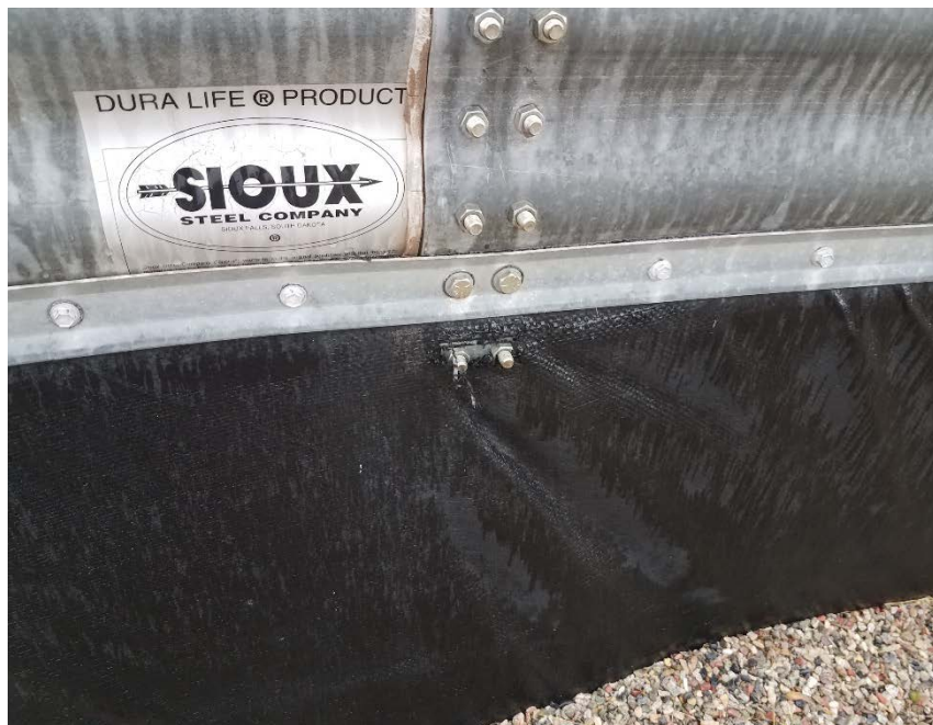
Location Photo #5, holes in secondary containment liner.
