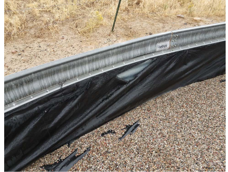
Location Photo #4, holes in secondary containment liner.
