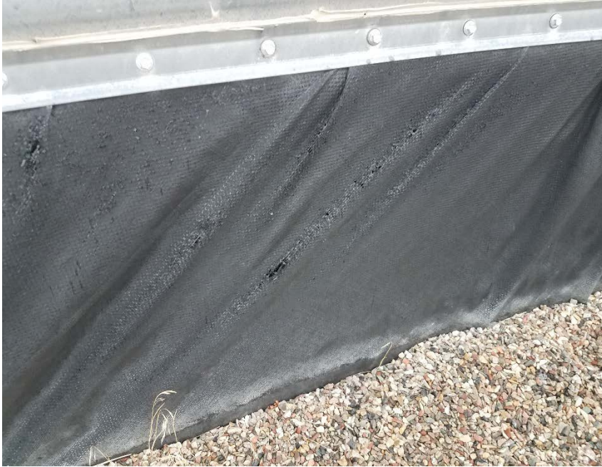
Location Photo #5, holes in secondary containment liner.
