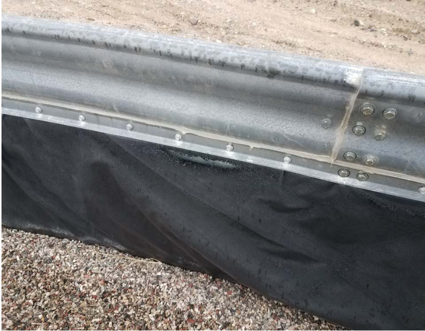
Location Photo #3, holes in secondary containment liner.
