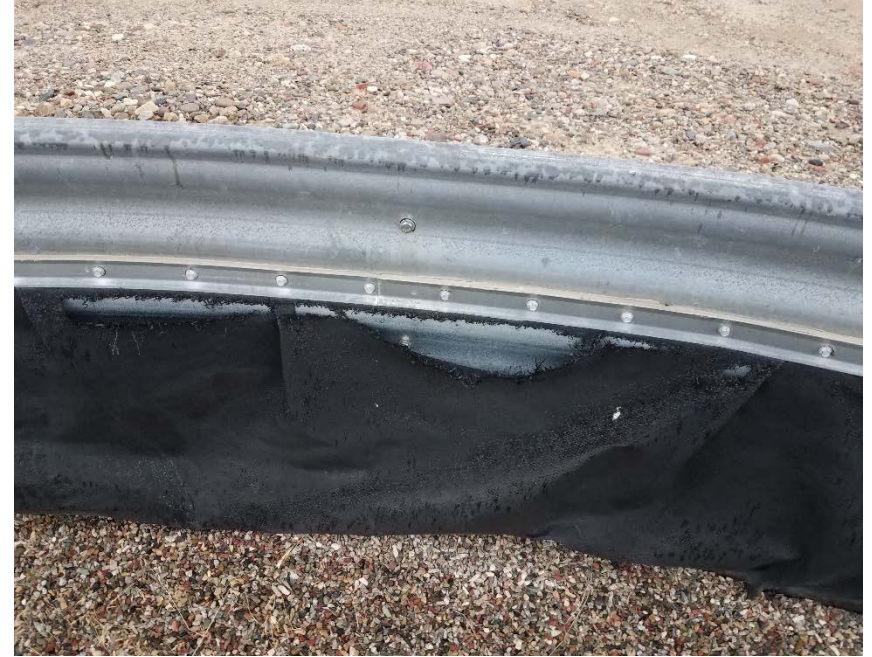
Location Photo #4, holes in secondary containment liner.
