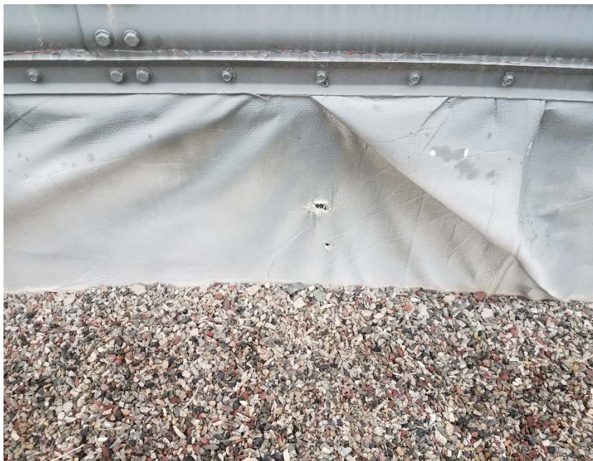
Location Photo #3, Holes in North battery liner.
