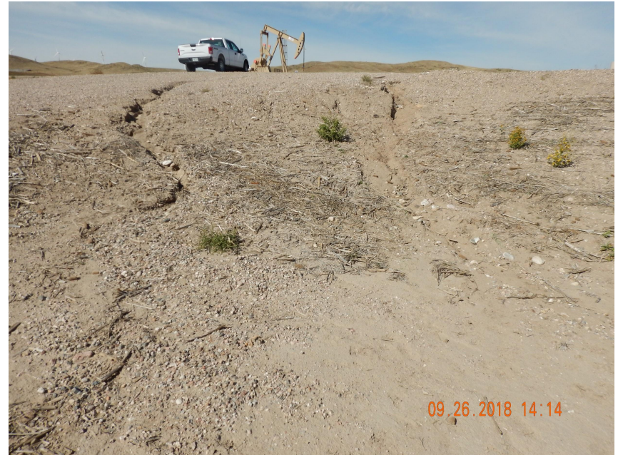
Photo 6. Photo taken from the southern location, facing North. Rill erosion forming along the southern fill slope. Stormwater repairs are required.
