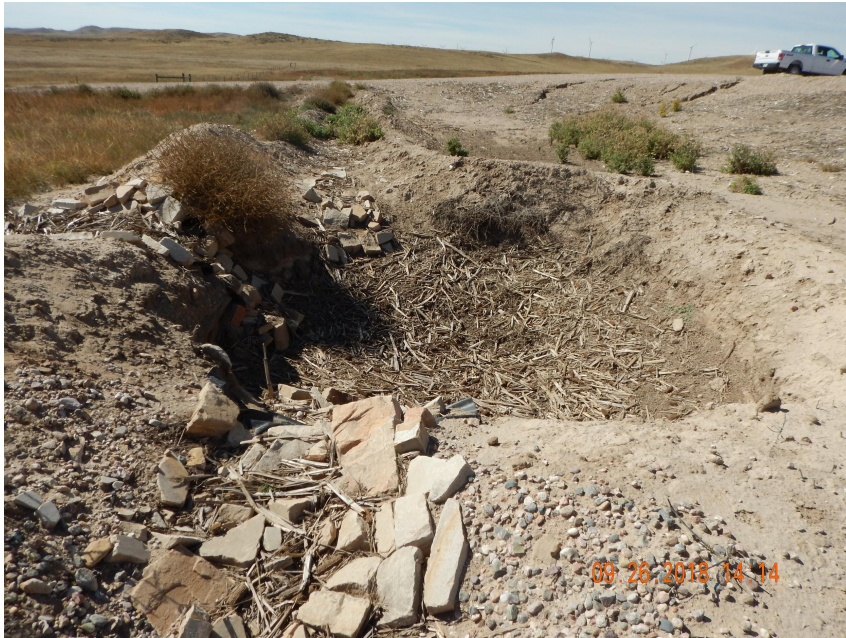
Photo 5. Photo taken from the southern location, facing West. Stormwater BMP maintenance is required as the sediment trap is not in proper functioning condition.
