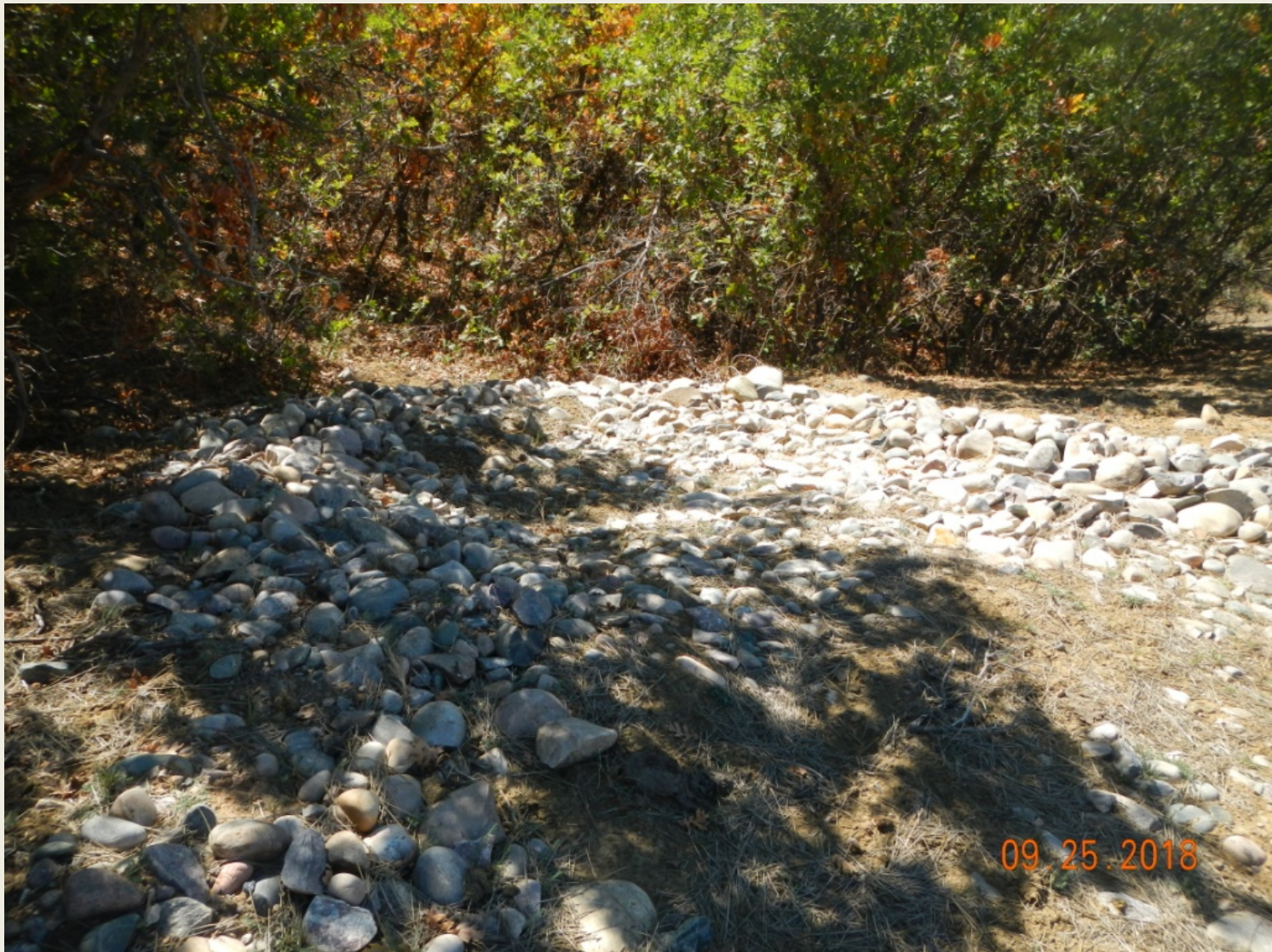
Photo 6. View of cobble run-down in the southeastern project area, appears to be functioning at this time.
