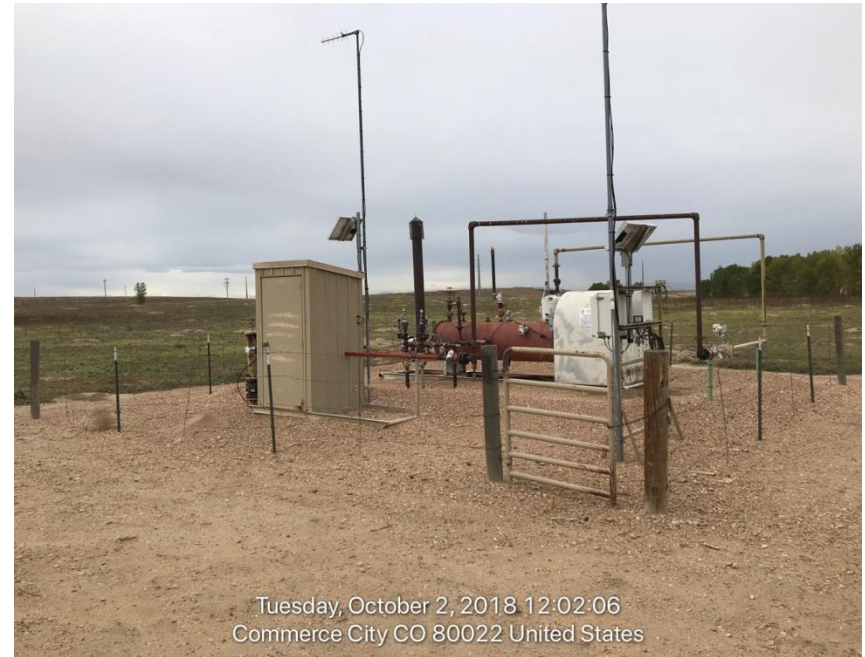
Photo#2 Separator and Gas Meter
