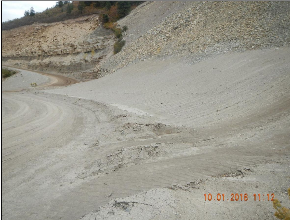
Tire traffic damaged berm.
