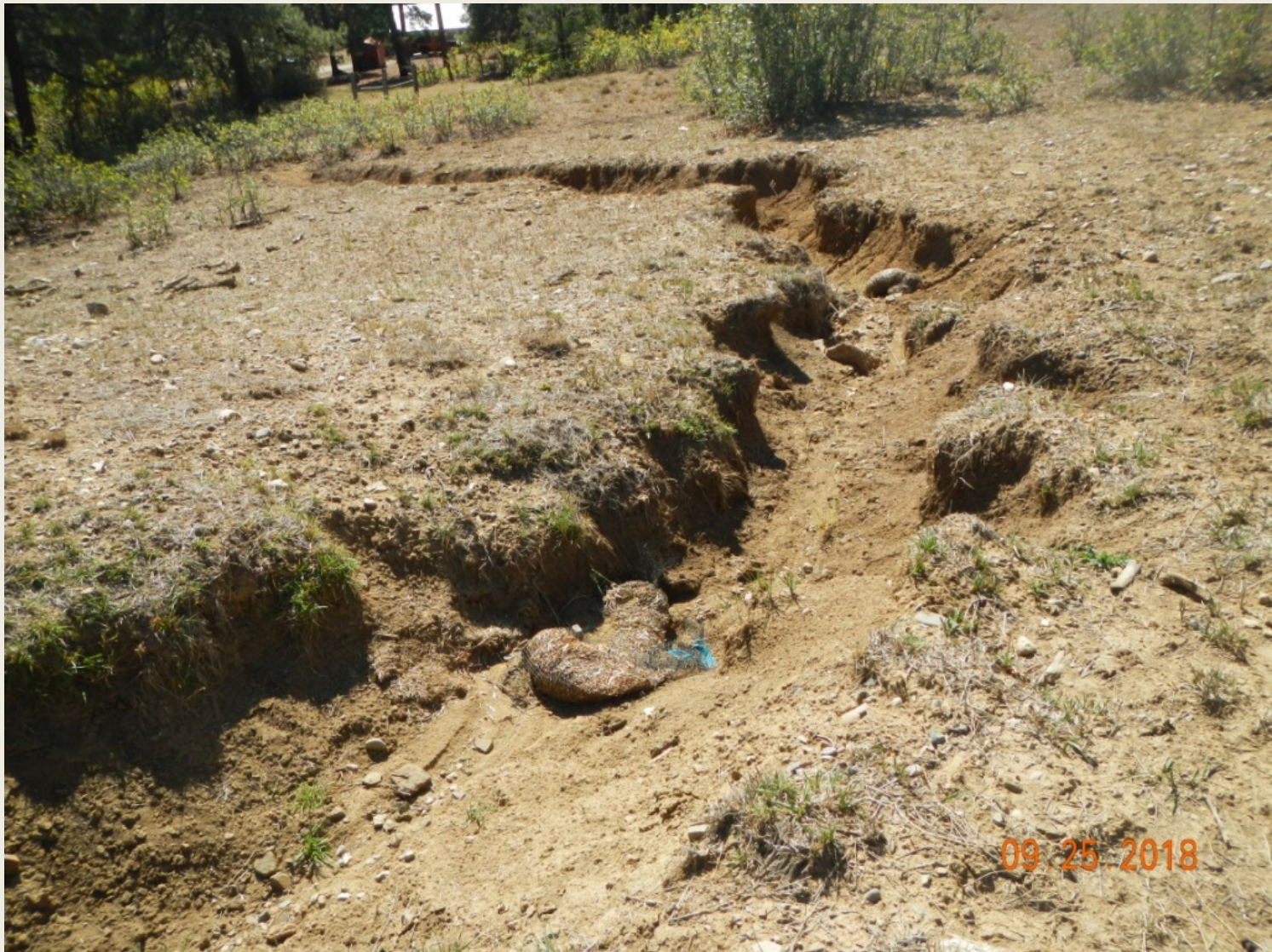
Photo 5. View of erosional channel up to 3 feet deep and 4 feet wide, in the southwestern project area. Wattles are not sufficient for stabilizing this portion of the project area.
