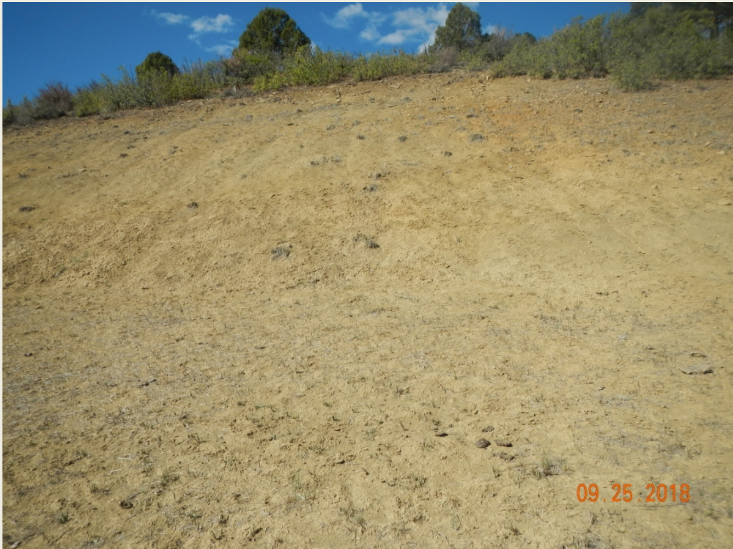
Photo 4. View of area on the western cut-slope with poor revegetation. This needs to be monitored and if revegetation is not progressing , the further seeding and reclamation efforts will be required.
