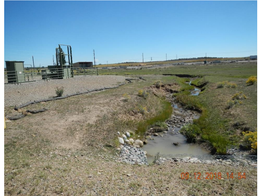
Wattles on western edge of location, along tributary of Rock Creek.
