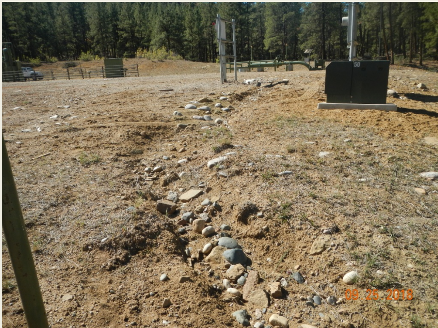
Photo 4. View of erosional channel approximately 15 inches deep and 24 inches wide in the northern project area.
