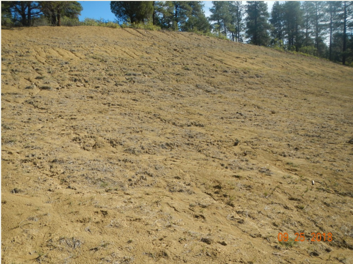
Photo 4. View of the northern cut slope from the central toe of slope facing up-slope. Vegetation is sparse and significant rilling/run-on is occurring.
