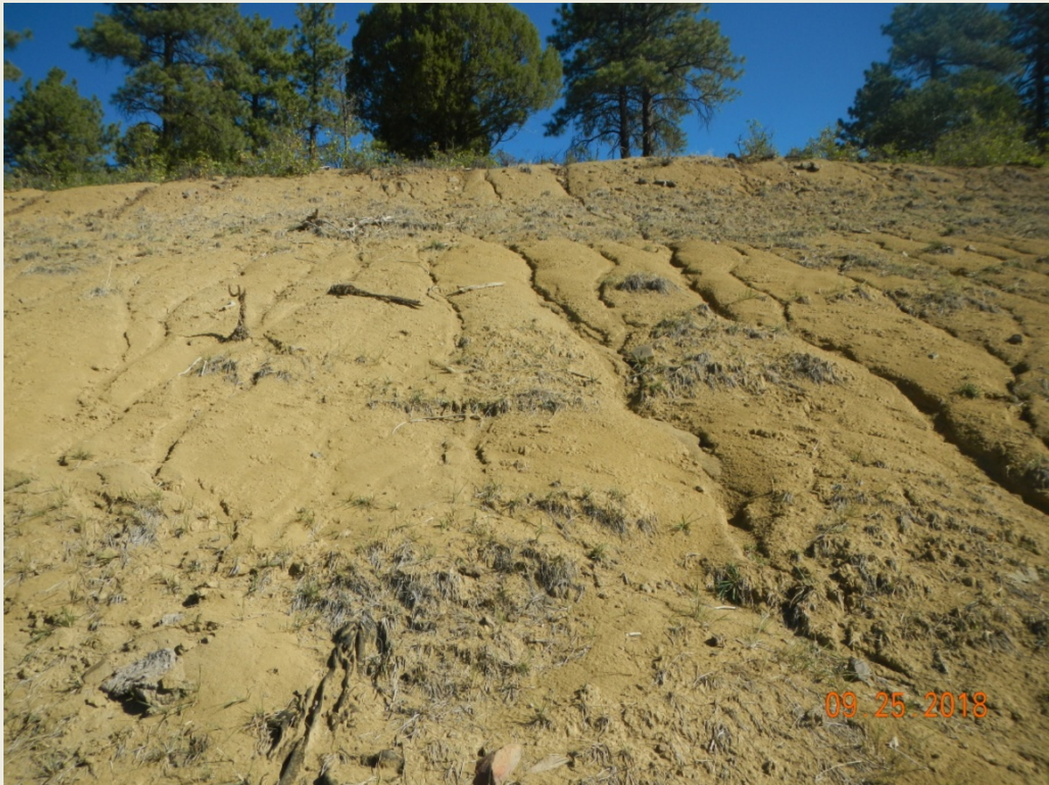
Photo 4. Closeup view of rilling on the northern cut-slope up to 10 inches wide and deep. Run-on controls, erosion controls such as erosion blankets, and cattle exclusion are likely needed to stabilize slope. Seeding is needed where vegetation is not becoming established.
