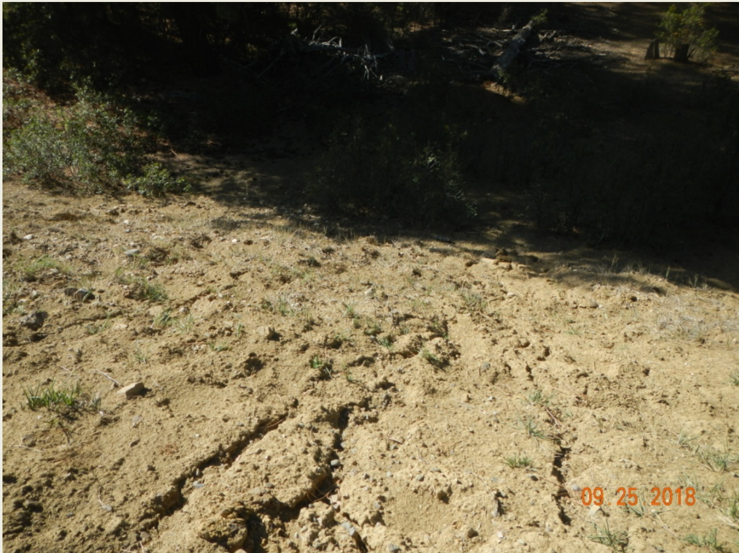
Photo 8. View of rilling in the southern cut-slope, facing down-slope.
