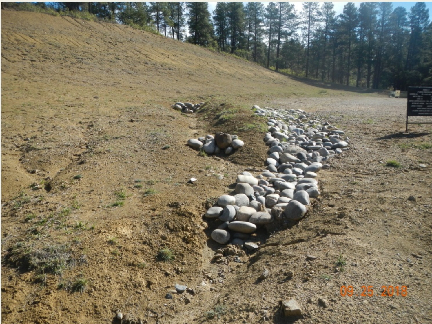
Photo 9. View of cobble armoring in the northwestern corner of the working area where stormwater is diverted off of the northern project area.
