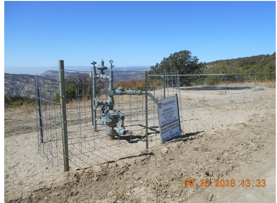
Wellhead with sign, blowdown pit in background
